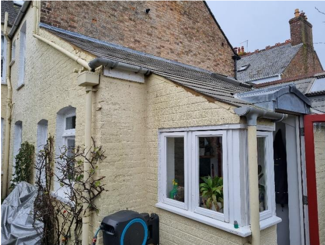
Photo 1: East facing elevation roof
