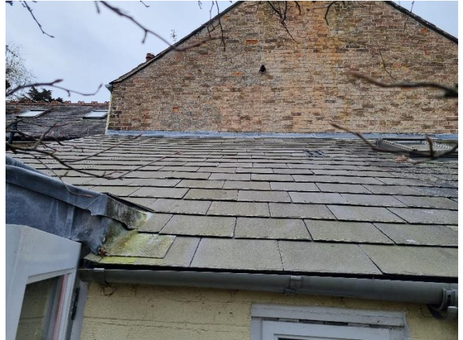
Photo 2: East facing elevation roof tiles
