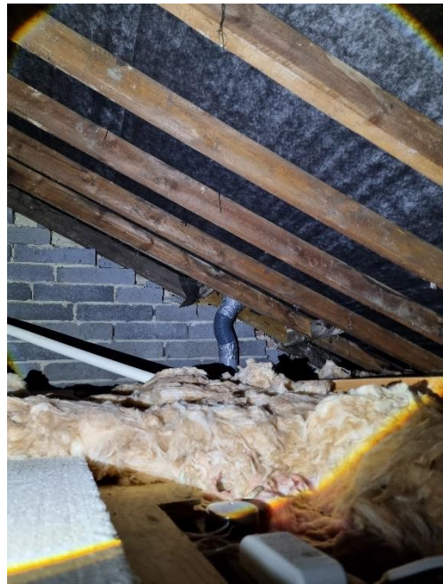
Photo 4: Loft void above existing extension
