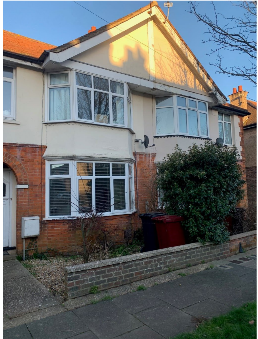
Photo 2-Front elevation of 34 Orchard Avenue, Chichester
