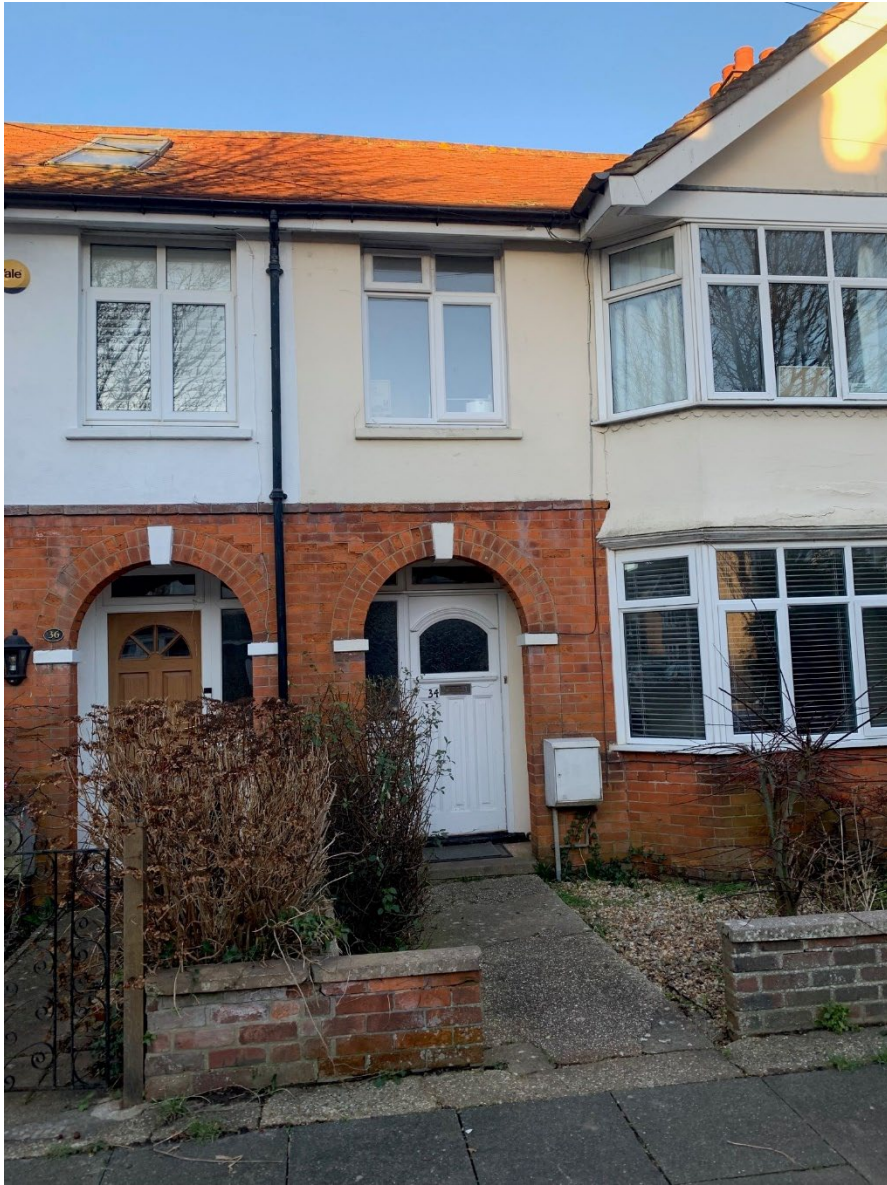
Photo1- Front elevation of 34 Orchard Avenue, Chichester
