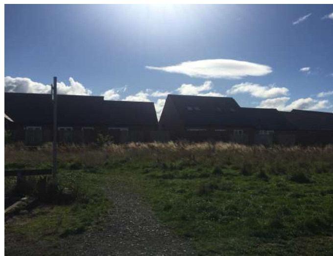
View across C2C to rear of adjacent bungalows.
