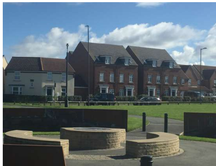
View East across Fawcett Park and C2C to adjacent housing.
