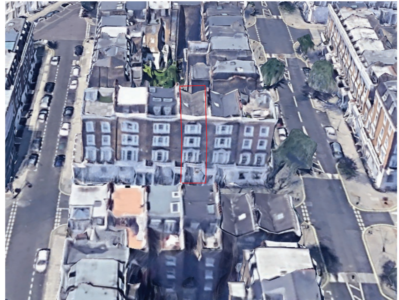
Aerial view of 42 Sussex Street_Front of building
