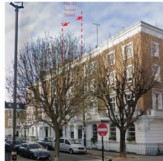
2). Site image looking west towards 42 Sussex Street
