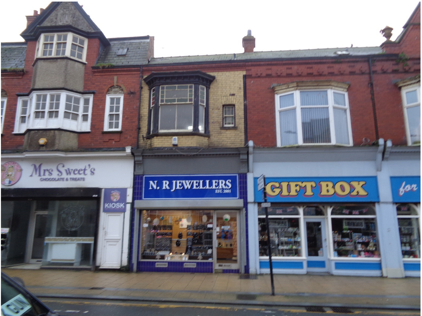
Figure 1: Roller shutter as installed.
