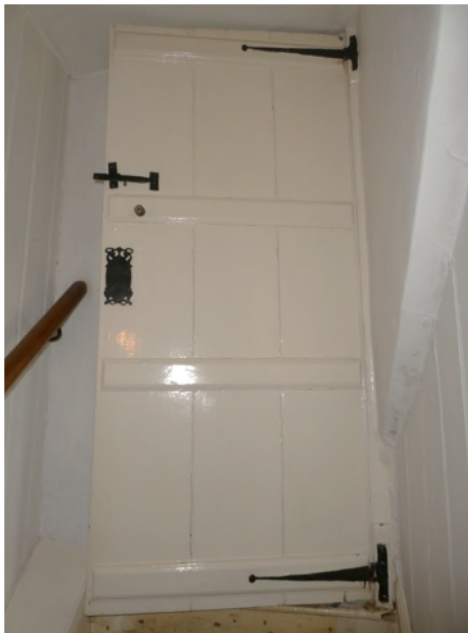
Figure 45: Plank and batten door to the room over the cellar
