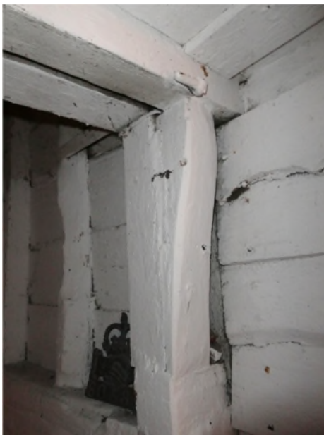
Figure 43: Reused timbers in the cellar
