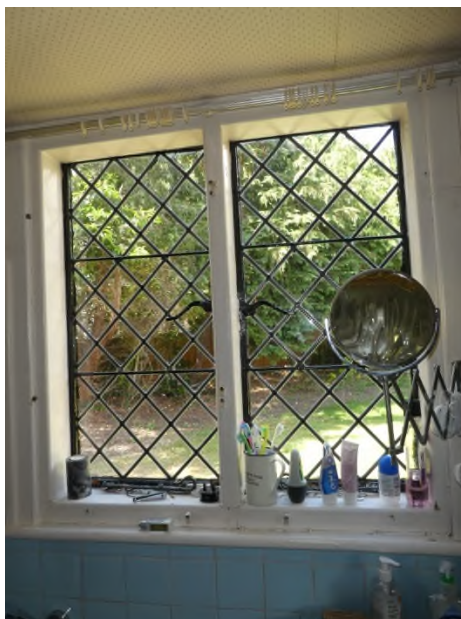
Figure 56: Late 19 th to early 20 th century leaded lights to be removed and retained on display within the building
