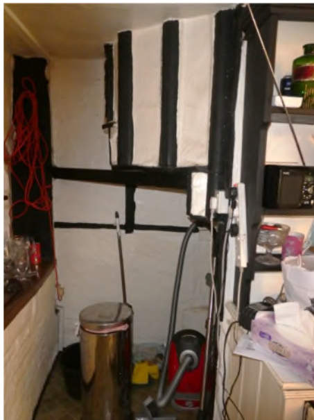
Figure 28: Stair enclosure in the kitchen
