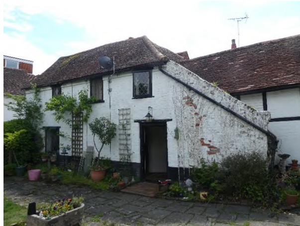
Figure 32: Parapeted outshut to the rear of Phase 3
