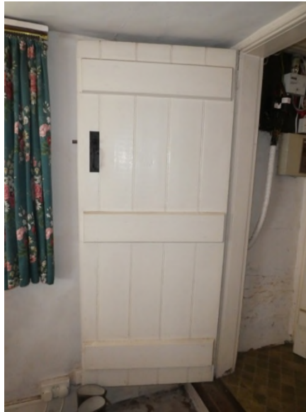
Figure 25: Late 19 th to early 20 th century plank and batten door to the dining room from the kitchen
