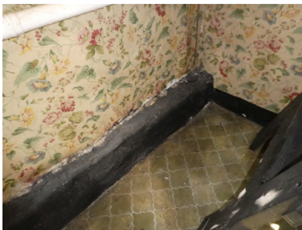
Figure 41: Sole plate on the south-western side of Phase 4
