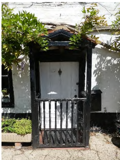
Figure 52: Existing porch on the south-west elevation
