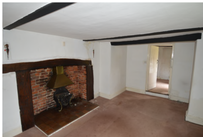
Figure 34: Brick fireplace with timber lintel
