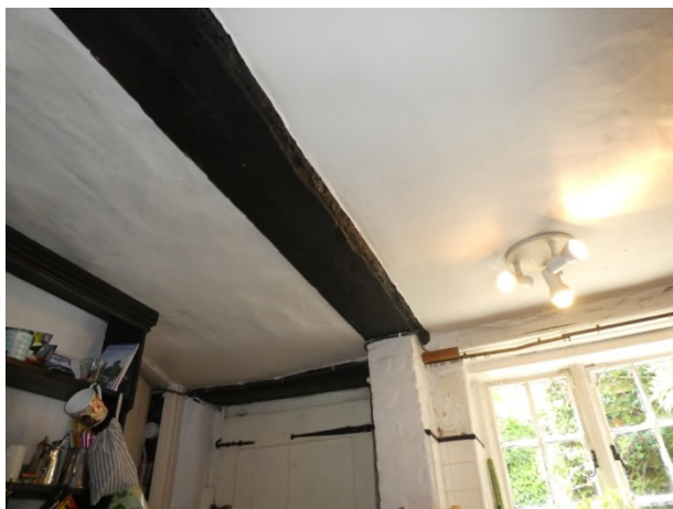
Figure 17: Axial beam in the south-west ground floor bay of Phase 1
