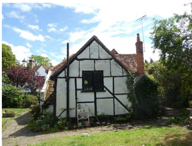
Figure 55: Gable end elevation of the Phase 5 extension
