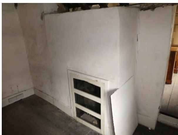
Figure 29: Fireplace in bedroom 1
