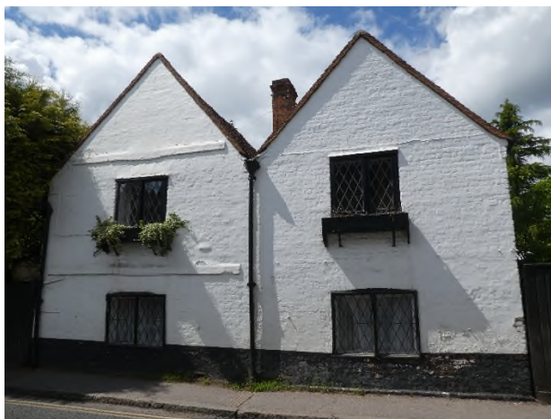
Figure 1: Front elevation of Old Timbers
