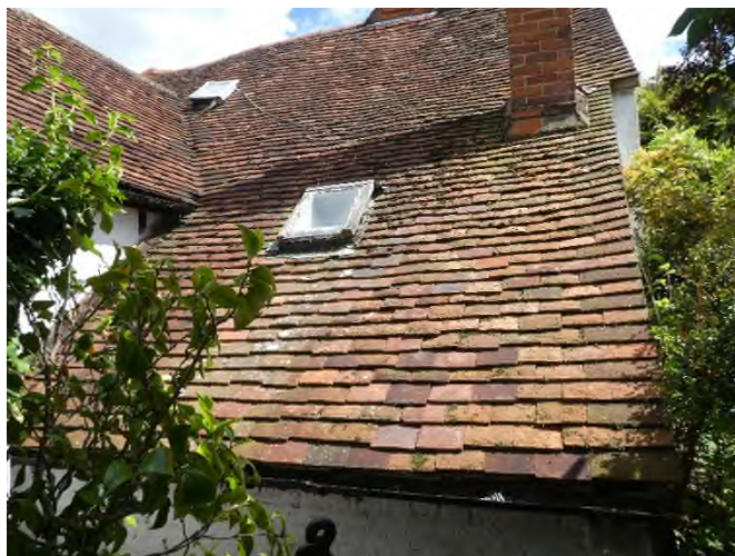
Figure 54: Existing rooflights to be replaced with more appropriate conservation rooflights
