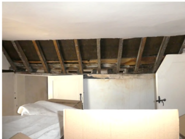
Figure 35: Exposed common rafters in bedroom 2
