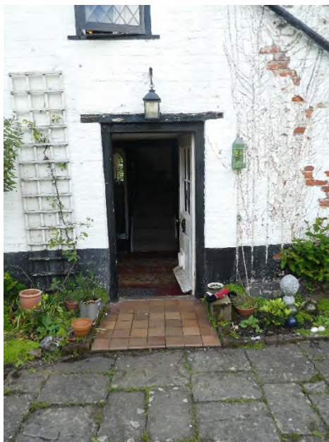
Figure 57: Existing door on the garden elevation
