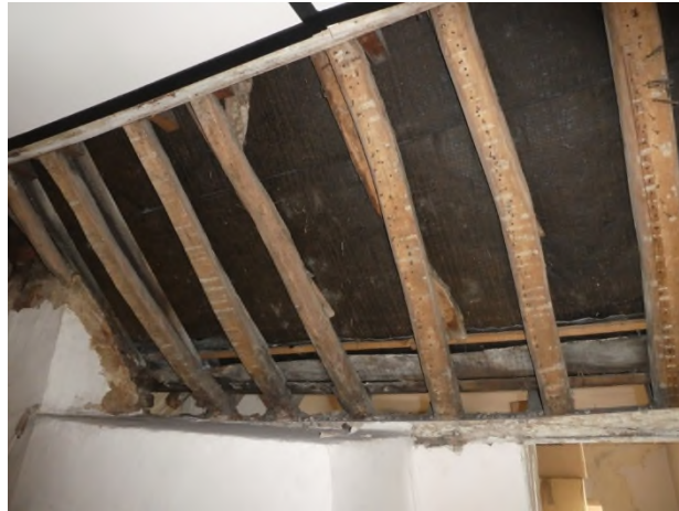
Figure 30: Exposed rafters above the chimney breast in bedroom 1
