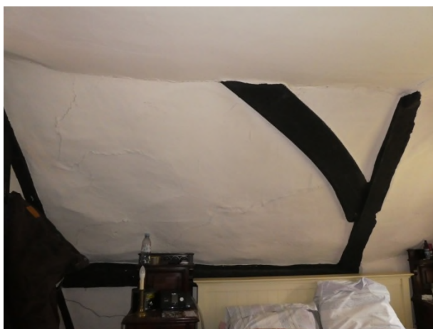
Figure 15: Curved windbrace in the northern corner of Phase 1
