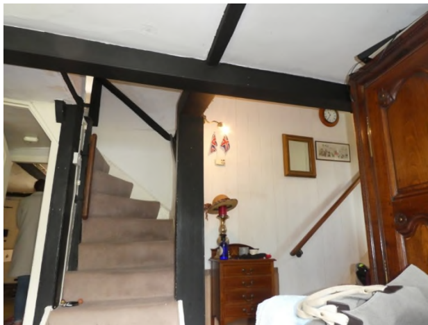
Figure 37: 20 th century beams and posts in the entrance hall
