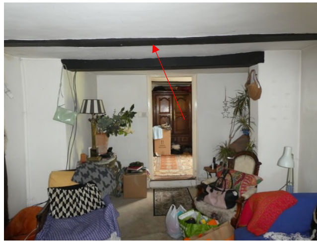
Figure 21: Beam in the living room that defines the south-east side of the north-east bay of Phase 1
