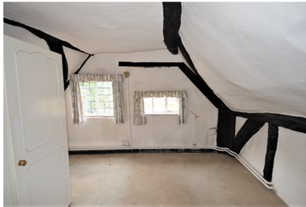
Figure 11: South-west gable end frame with curved windbrace to left of photo
