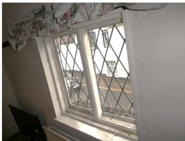
Figure 50: Modern leaded lights within an earlier frame in the bedroom
