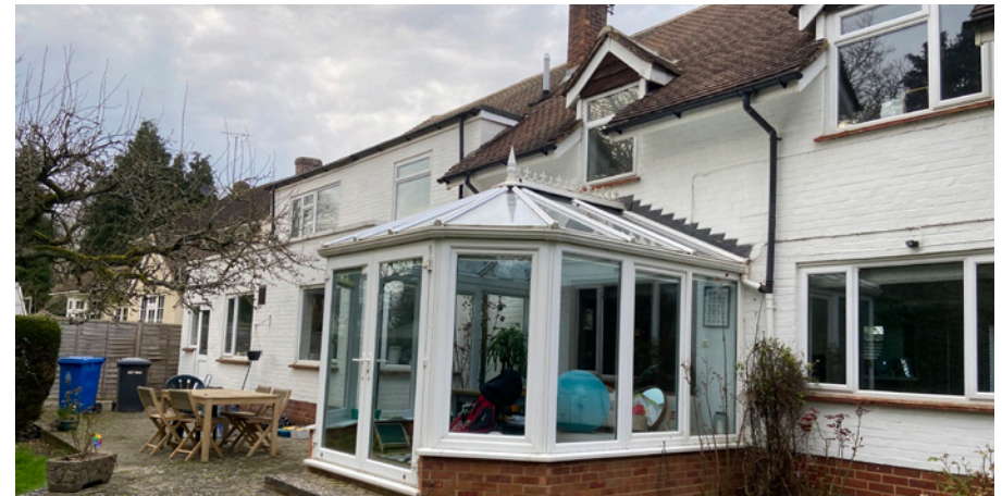
Fig. 03 View of the rear of the property
