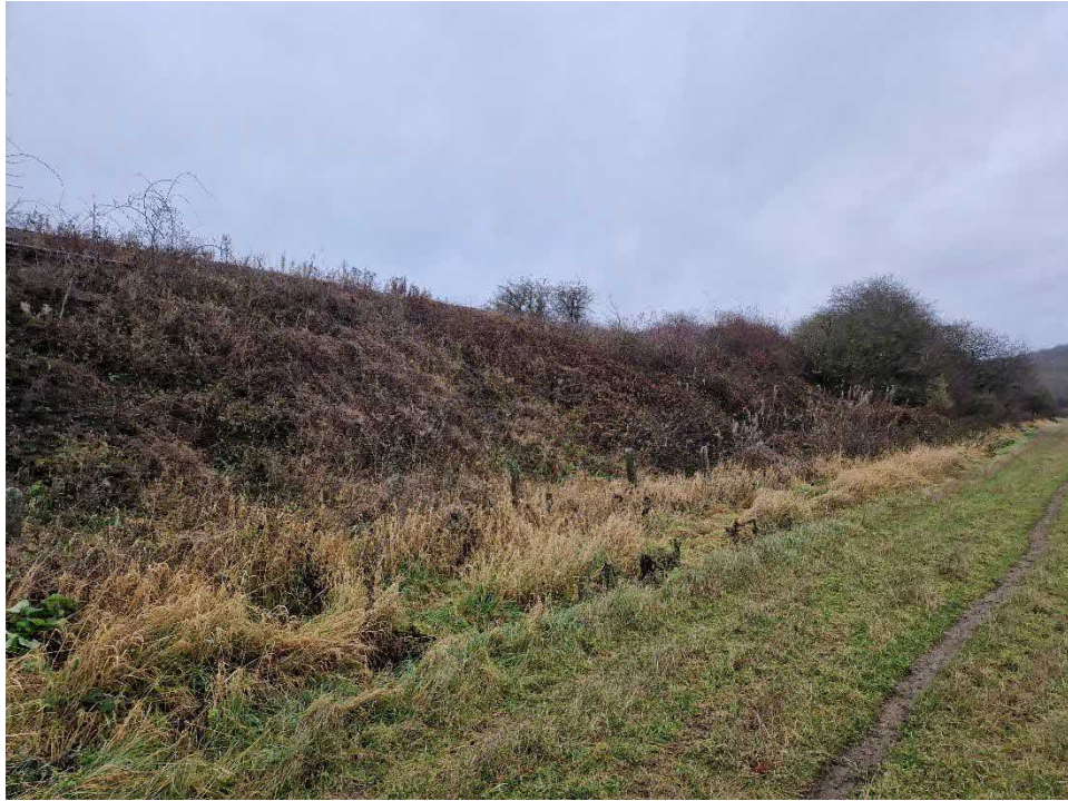
Plate 4-7 - Railway line that runs along the northern boundary of the site, facing north-east (WSP, 2023)
