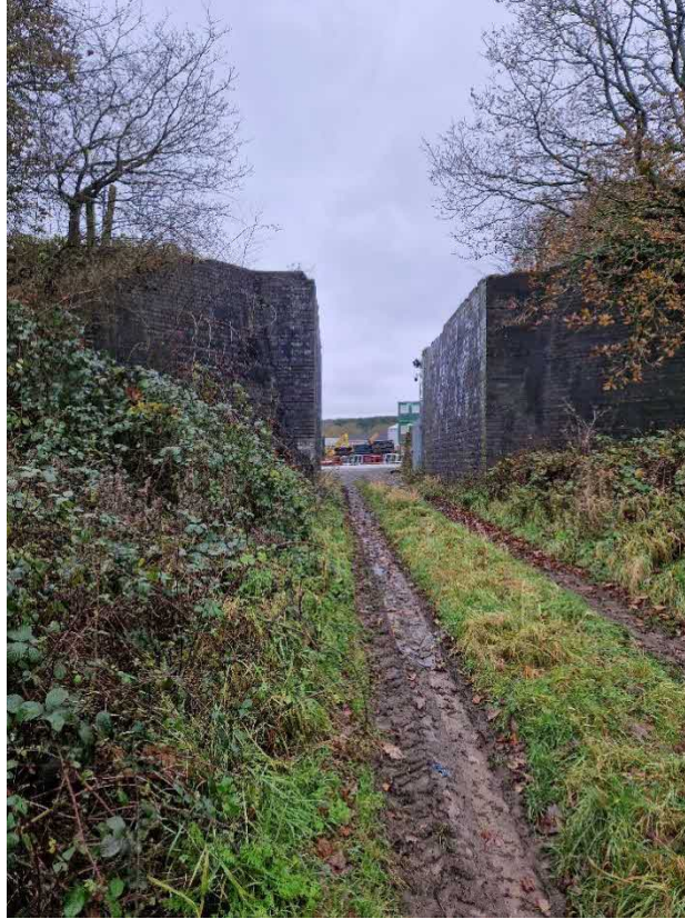
Plate 4-11 - Railway bridge and trackway leading from the fields to the Murphy's Plant Ltd complex, facing south-west (WSP, 2023)
