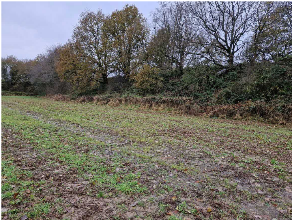
Plate 4-10 - Embankment of the railway line in the central part of the site, facing south-west (WSP, 2023)
