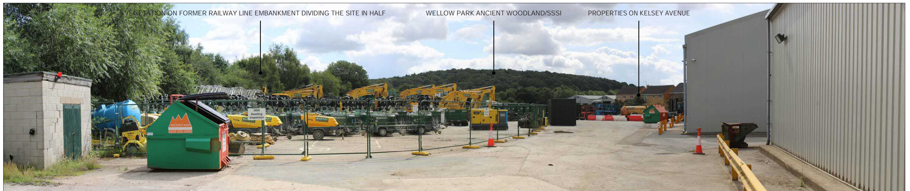
PHOTOGRAPH –VIEWPOINT S2 VIEW FROM THE NORTHERN EDGE OF THE JMS SITE, LOOKING SOUTH EAST TOWARDS WELLOW PARK, WHICH IS VISIBLE ON THE HORIZON. PROPERTIES ON KELSEY AVENUE ARE VISIBLE ADJACENT TO THE SITE BOUNDARY. VIEWS OF THE EASTERN HALF OF THE SITE ARE TRUNCATED BY THE VEGETATED FORMER RAILWAY LINE EMBANKMENT.
