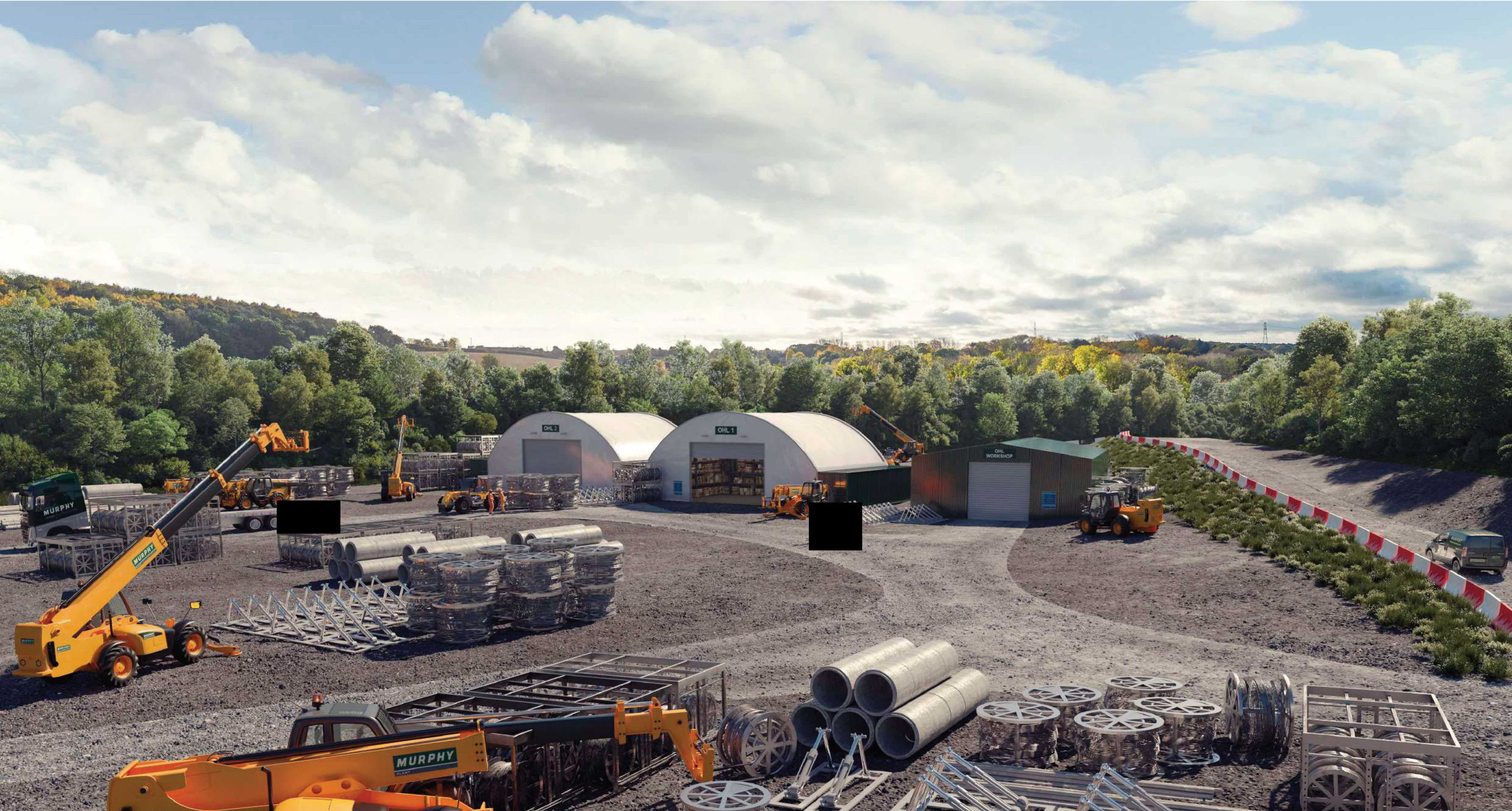
View south towards storage buildings and OHL workshop
