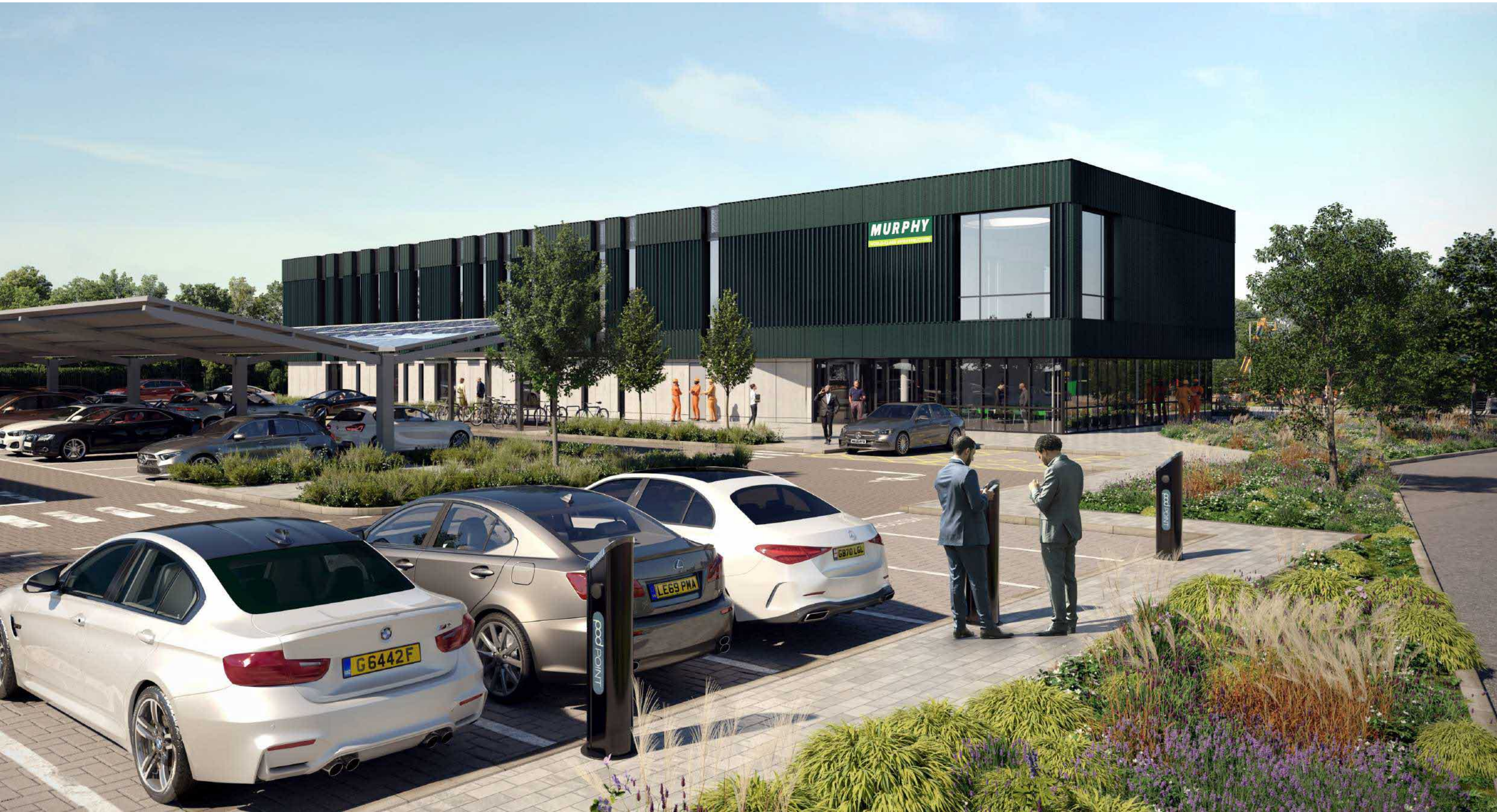
View east towards the office and training building
