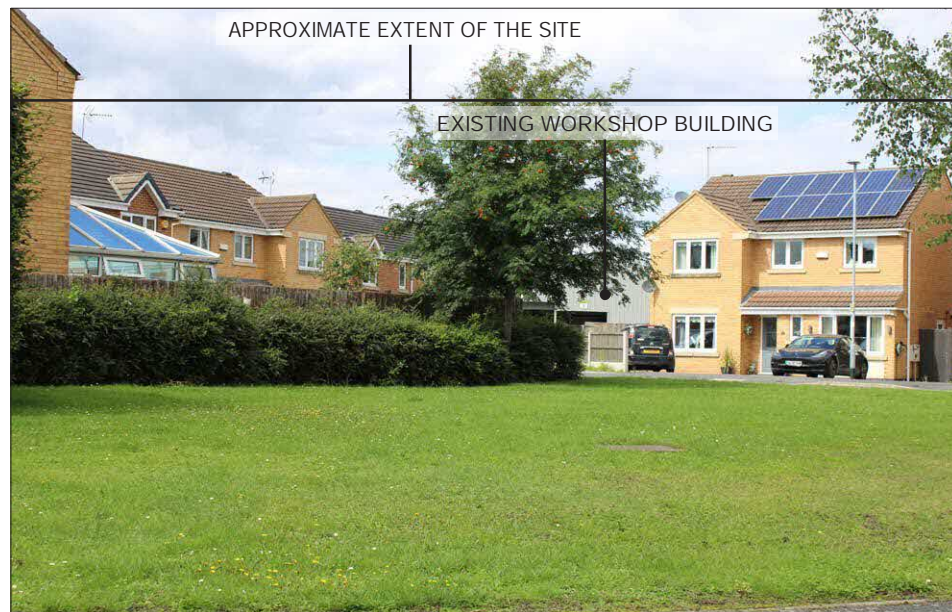
PHOTOGRAPH –VIEWPOINT 9 VALUE: LOW VIEW FROM KELSEY AVENUE, LOOKING NORTH TOWARDS THE SITE, THERE ARE PARTIAL VIEWS OF THE WORKSHOP BUILDINGS BETWEEN THE RESIDENTIAL PROPERTIES.
