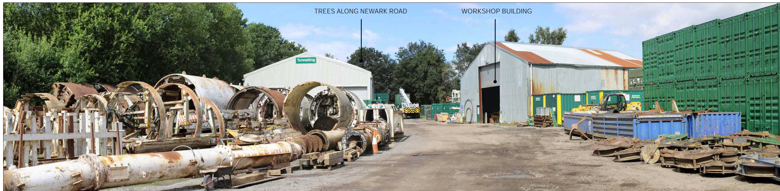
PHOTOGRAPH –VIEWPOINT S13 VIEW FROM THE SOUTH WESTERN PART OF THE JMS SITE, LOOKING WEST TOWARDS NEWARK ROAD. THE WORKSHOP BUILDINGS, CONTAINERS AND MACHINERY CREATE A SENSE OF ENCLOSURE AGAINST THE WOODED BACKDROP OF THE SITE BOUNDARIES.
