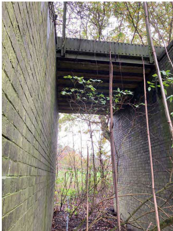
Photograph 10 – Bridge at the southern Site boundary
