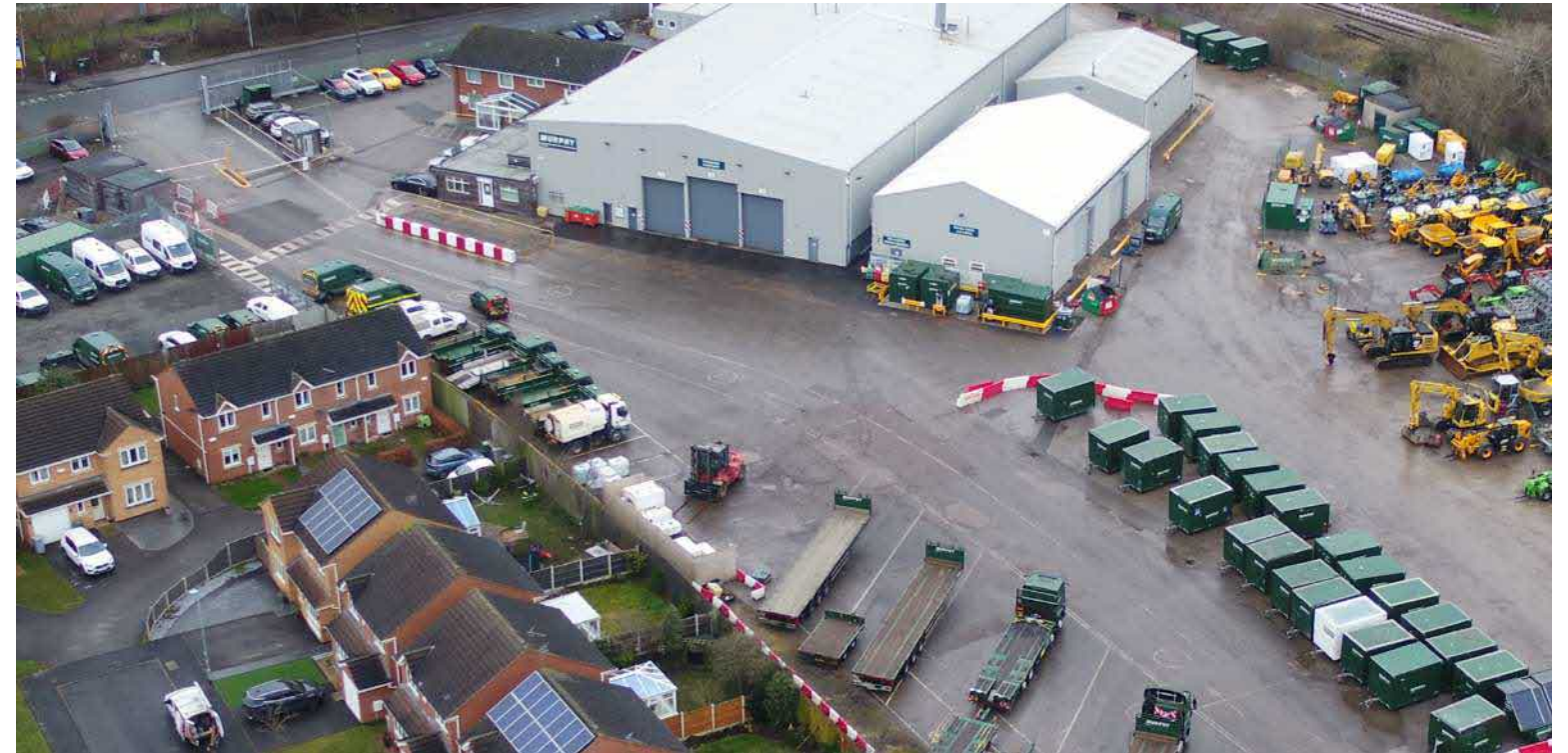
Drone image: Existing relationship between Kelsey Avenue and Murphy site entrance
