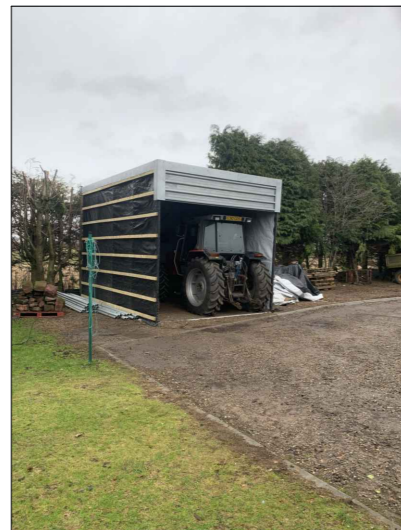
Existing Open Shed to be removed
