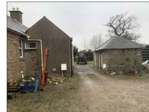
Existing Outbuilding to be removed in relation to Cottage
