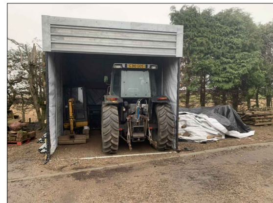
Existing Open Shed to be removed
