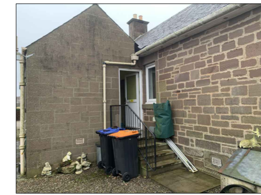
Part Cottage South-West Elevation
