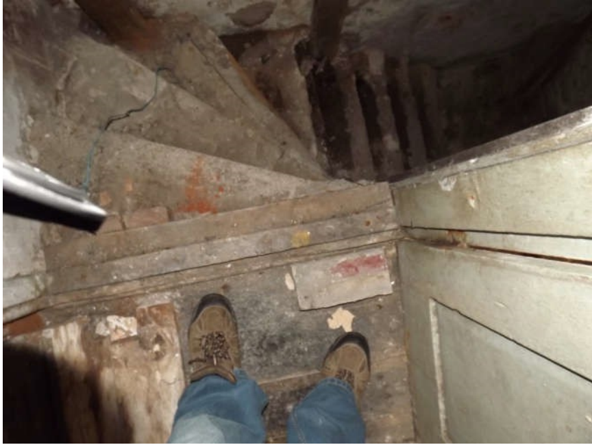
Cellar Stairs Down
