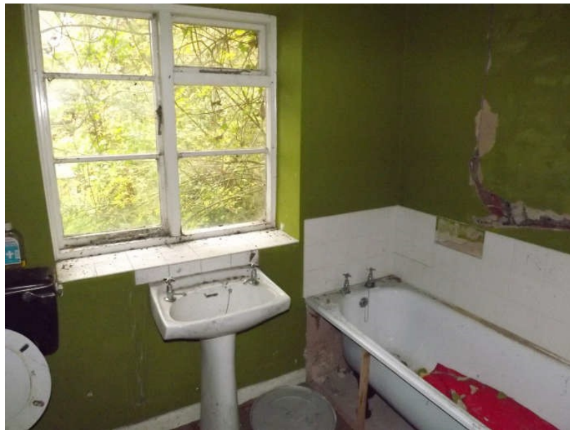
Ground floor bathroom.
