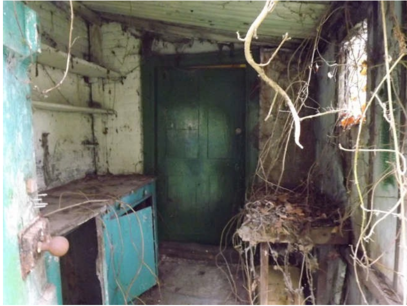
North elevation east facing 'Porch' No 9
