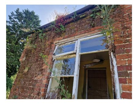
In the current condition, underpinning which has been approved to address the subsidence has an exceedingly high probability of causing collapse of the structure due to its weakened structural
