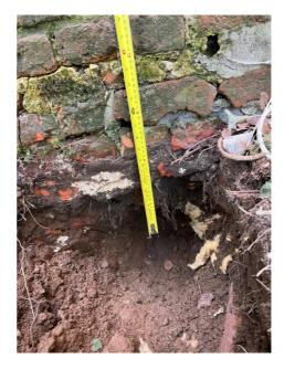
The lean-to does not have a damp course membrane, consequently the lower-level bricks are saturated with excess moisture causing spalling, evidenced by extensive flacking, and crumbling of the bricks. The spalling has damaged structural integrity, with parts of the brick & mortar falling off.
