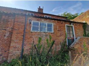
The internal floor level of the western section (b) is the same level as the main building, however, eastern section floor level Is 420mm lower than the main building and is falling down due to the absence of footings; it has slipped north down the hill breaking away from the main building with a gap of about 150mm and the floor to the east inside is subsiding such that the floor is out of level, also the earth/tile structure of the floor will endure the process of repairs.
