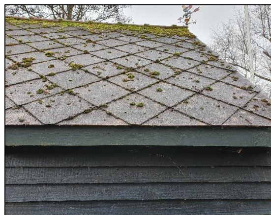
Figure 8: Outbuilding well fitted tiles and boarding.
