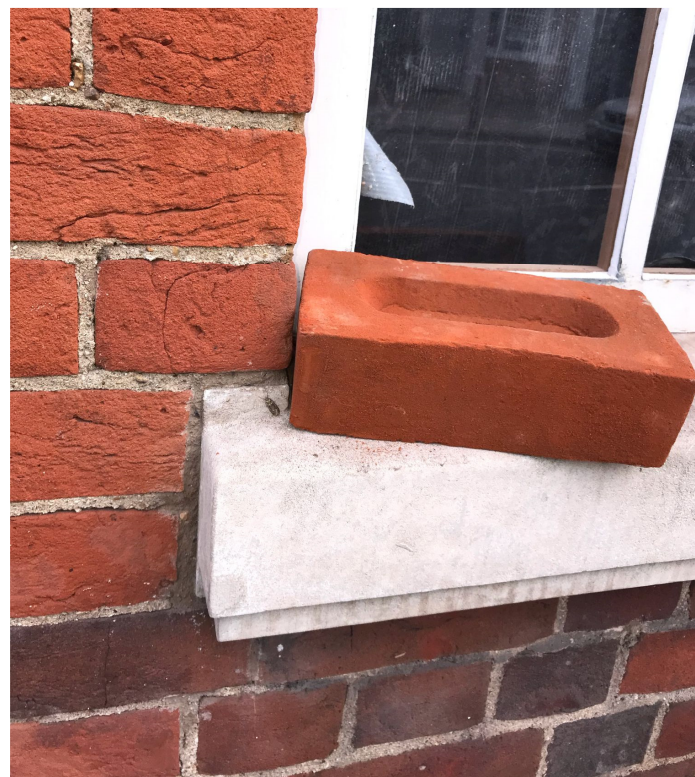
2. Proposed window surround detail brick
