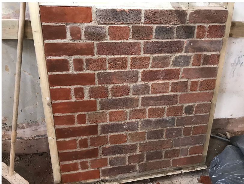
1. Sample Panel(photo taken internally)
