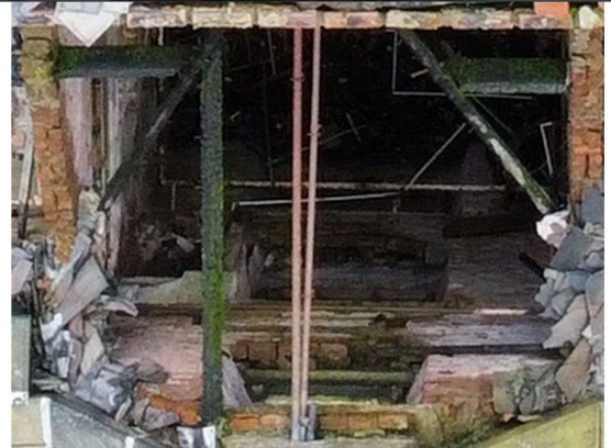
Rear centre room – remove fire-damaged timbers and loose material.
