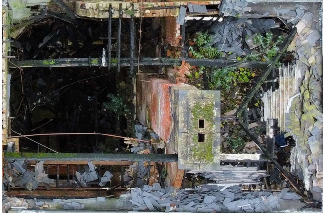
Rear centre room – remove fire-damaged timbers and loose material.
