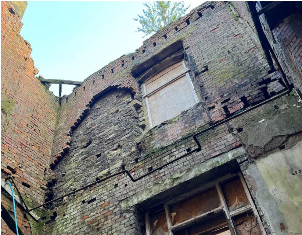
Photo 1, Room F3 Rebuild brickwork to support brickwork above.
