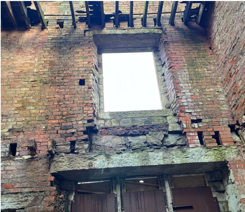
Room F9, rebuild brickwork under window.
