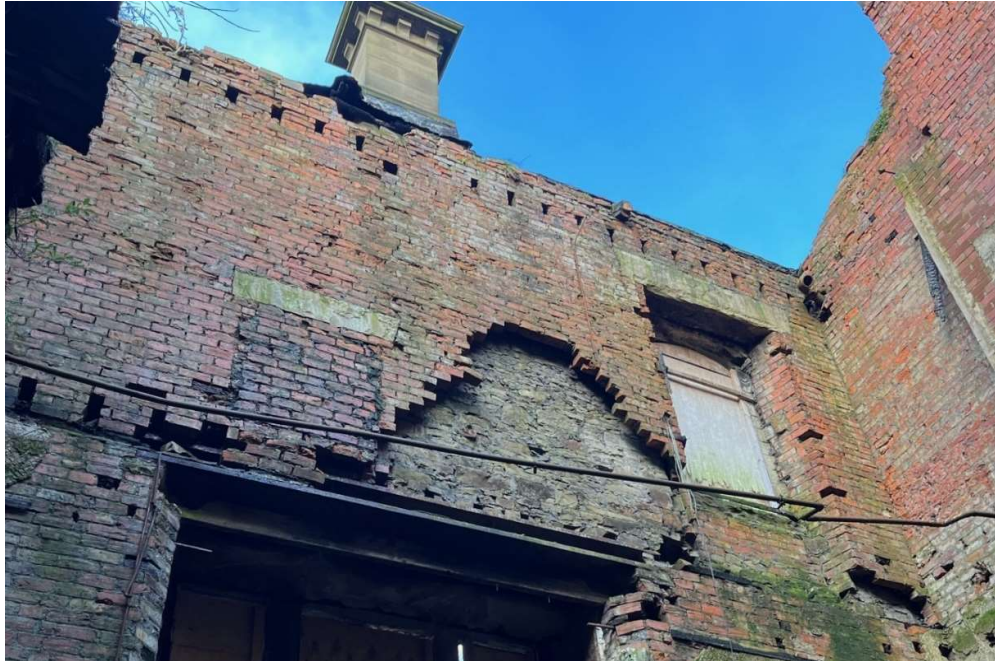
Photo 2 Room F1 Rebuild brickwork to support brickwork above.
