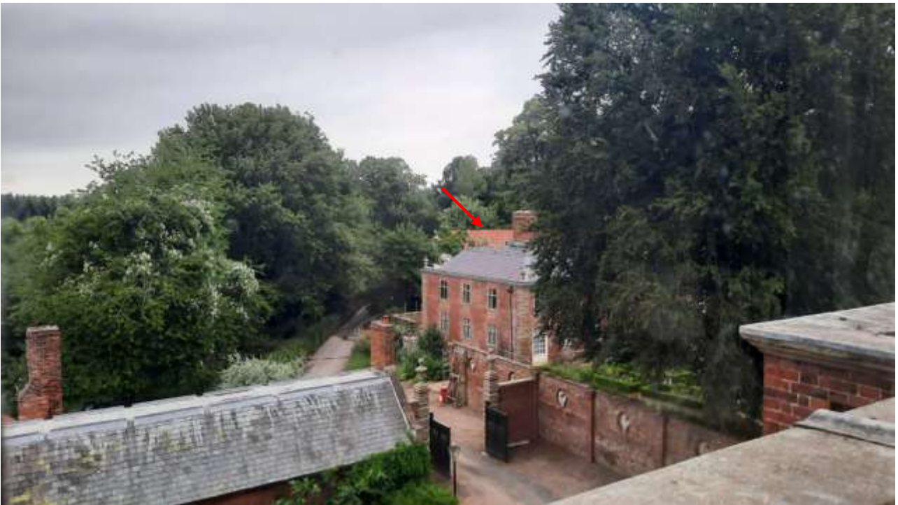
Fig. 4: View from the Main House second floor bathroom in the centre of the north elevation (window WS15) (red arrow points towards roof ducts)
