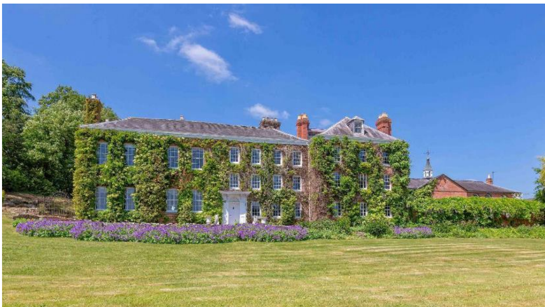
FIG 10 – Photograph of front elevation in summer, note soil stack almost invisible (Savills)
