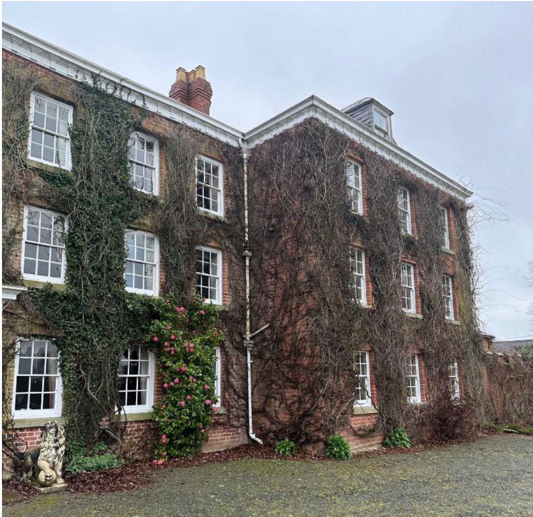
FIG 9 – Photograph of the front elevation from the southern aspect, note pipe now visible in Winter
