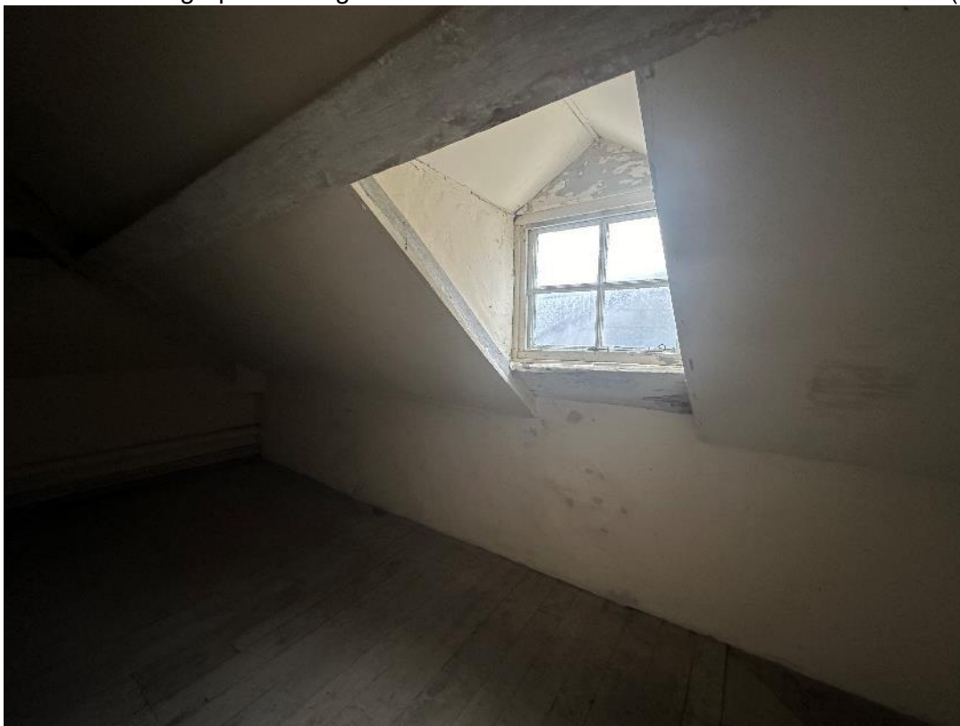
FIG 14 – Photograph of attic dormer to be enlarged (S Pemble)
