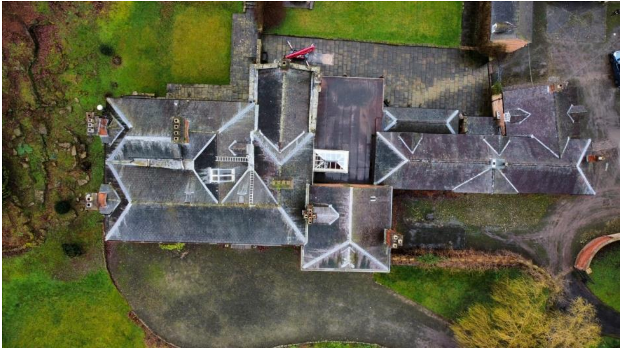
FIG 7 – Aerial photograph showing general roofscape of house (S Pemble)
