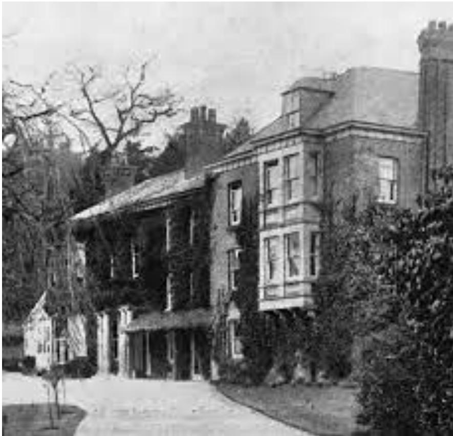
FIG 4 – Historic photograph of principal elevation, assumed early 20thC showing oriel bay and other additions no longer extant (Gareth Williams)
