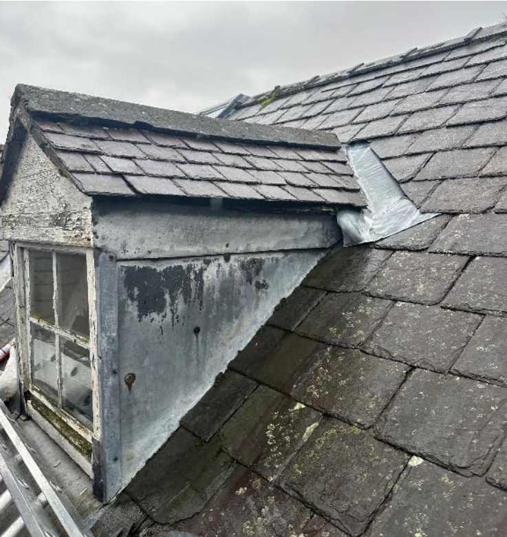
FIG 12 – Photograph of existing dormer to be enlarged (S Pemble)
