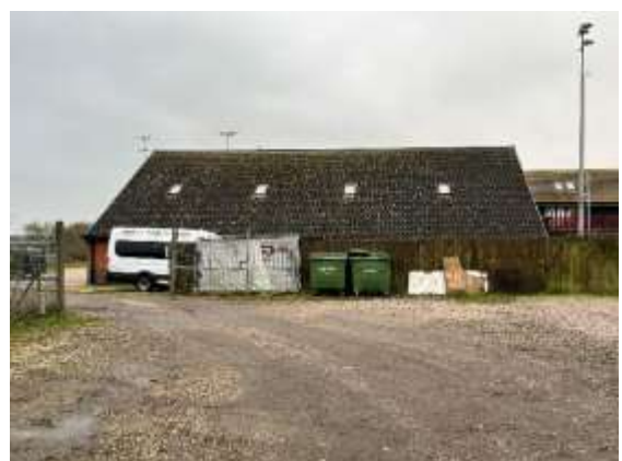
View from overspill carpark (North West elevation of existing clubhouse in background)
