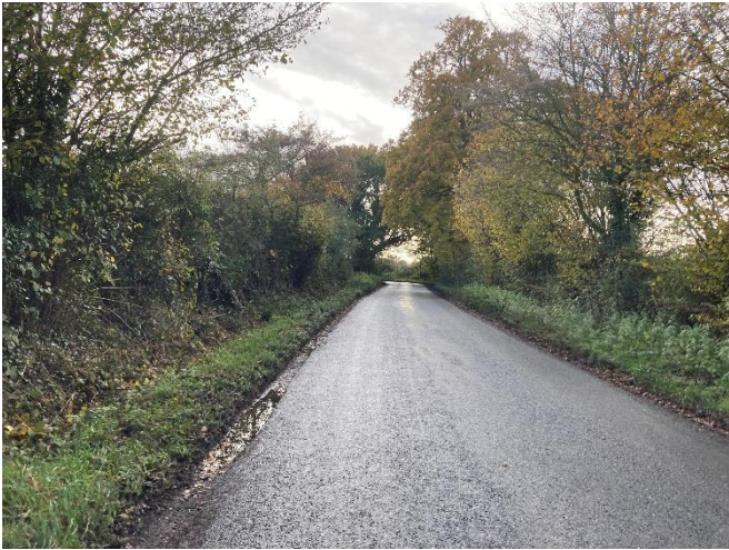
Typical view of boundary road and ditch with no water
