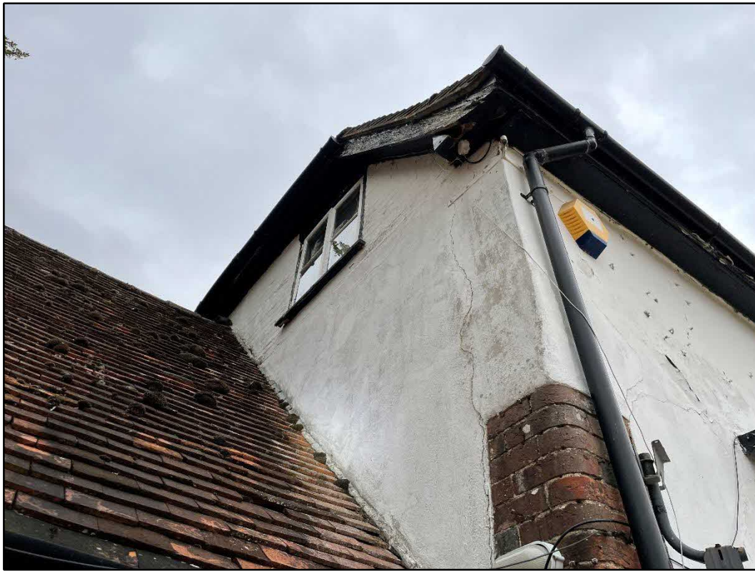
Plate 6. Locations of gaps at roof tiles and lead flashing
