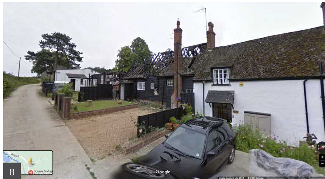
Figs 1-6: Interior photos of the Cottage and garages Figs 7-8: Previous buildings adjoining the Cottage, viewed from the private access lane, to the north-west (images courtesy of Google Maps during 2011)
