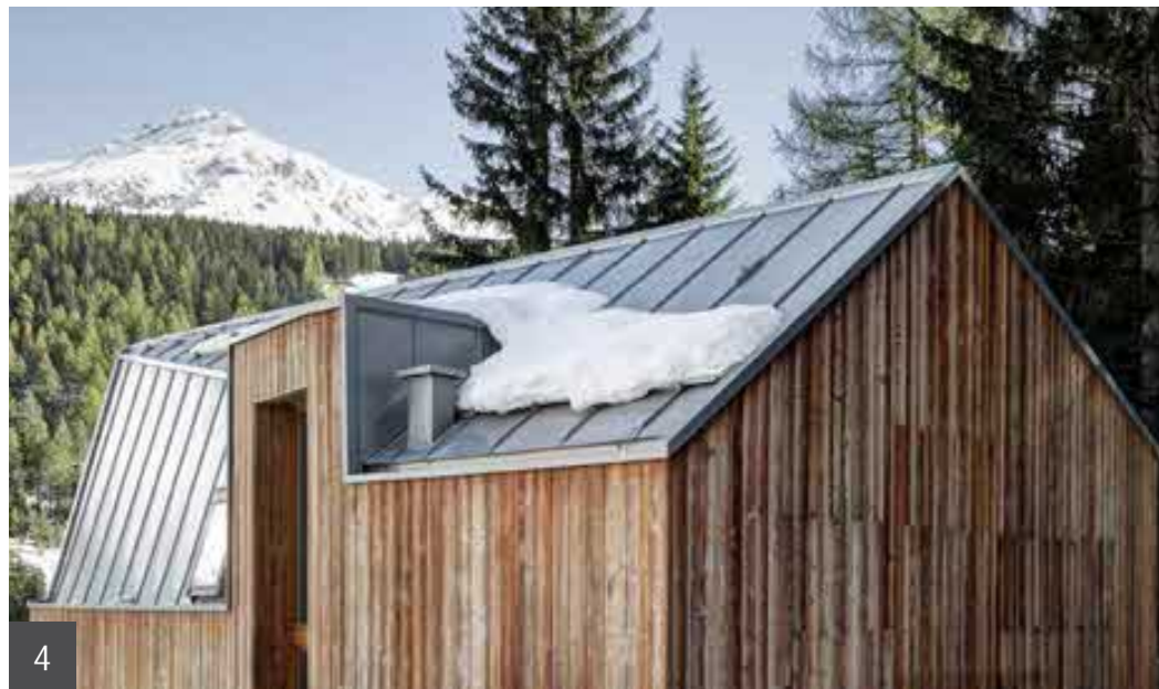
Fig 1-6: Timber clad building examples with contemporary glazed openings / detailing plus examples with standing seam roofs
