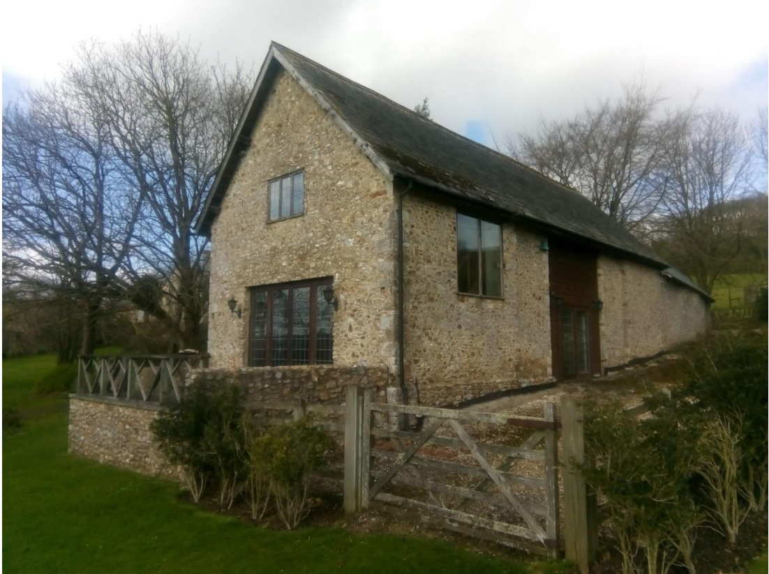
Photo of Building from the South East
