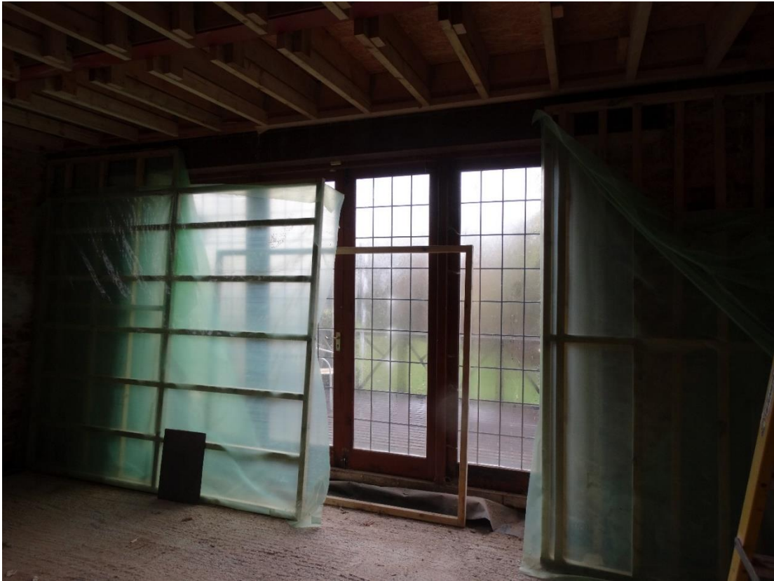
Current view looking south towards external decking area.
