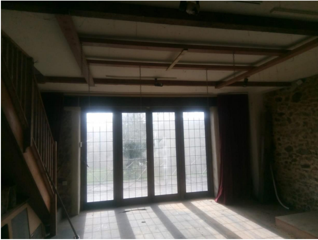
Looking South from inside the Area
