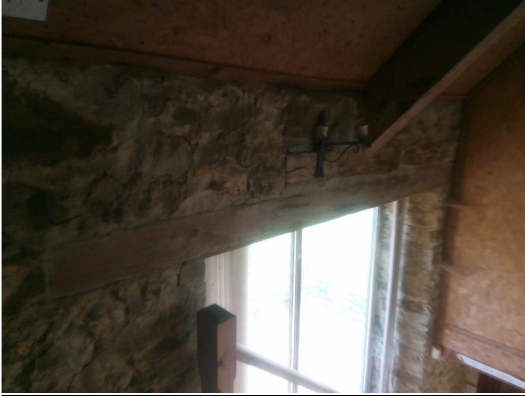
Original timber lintel over East window of Area
