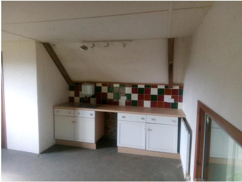
“Existing” Kitchen on First floor of Area now removed and forming part of a recent “retrospective” LBC application.
