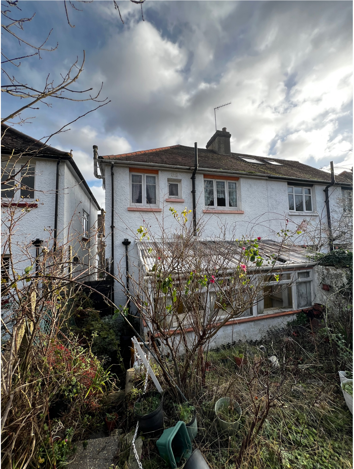
84 Ermine Road rear elevation
