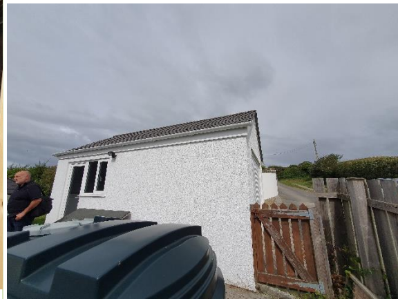
South aspect of separate garage building
