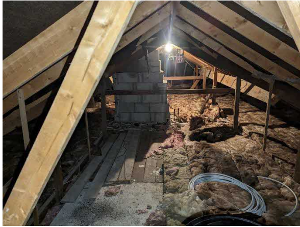
Photo 4. Showing the roof void over the eastern arm of the building
