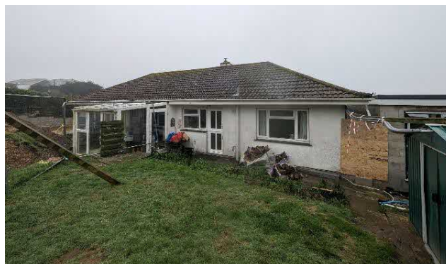
Photo 3. Showing the house from the rear
