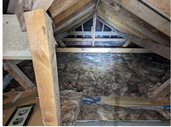
Photo 5. Showing the roof void over the southern arm of the building
