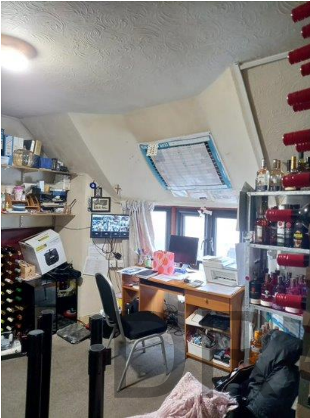
Plate 10. AB1 upstairs room, showing some original roof pitch#
