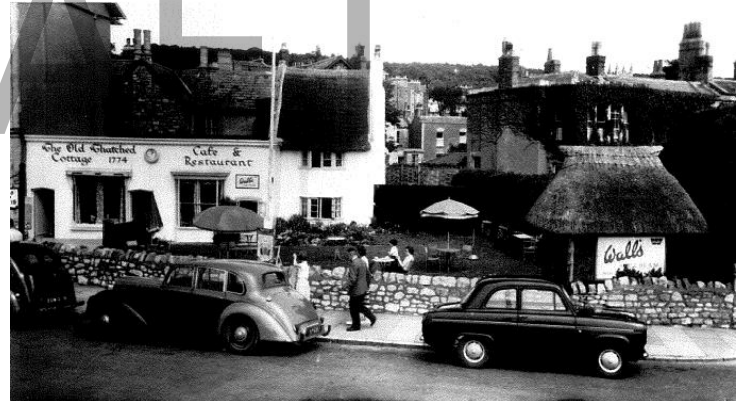
Figure 12. Photograph of the AB as the Thatched Cottage Restaurant in the 1950s.
