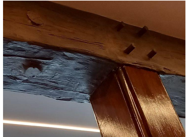
Plate 14. Beam in AB2 with apparent cladding
