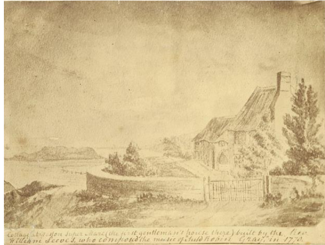
Figure 7. Illustration showing the original setting of Leeves Cottage
