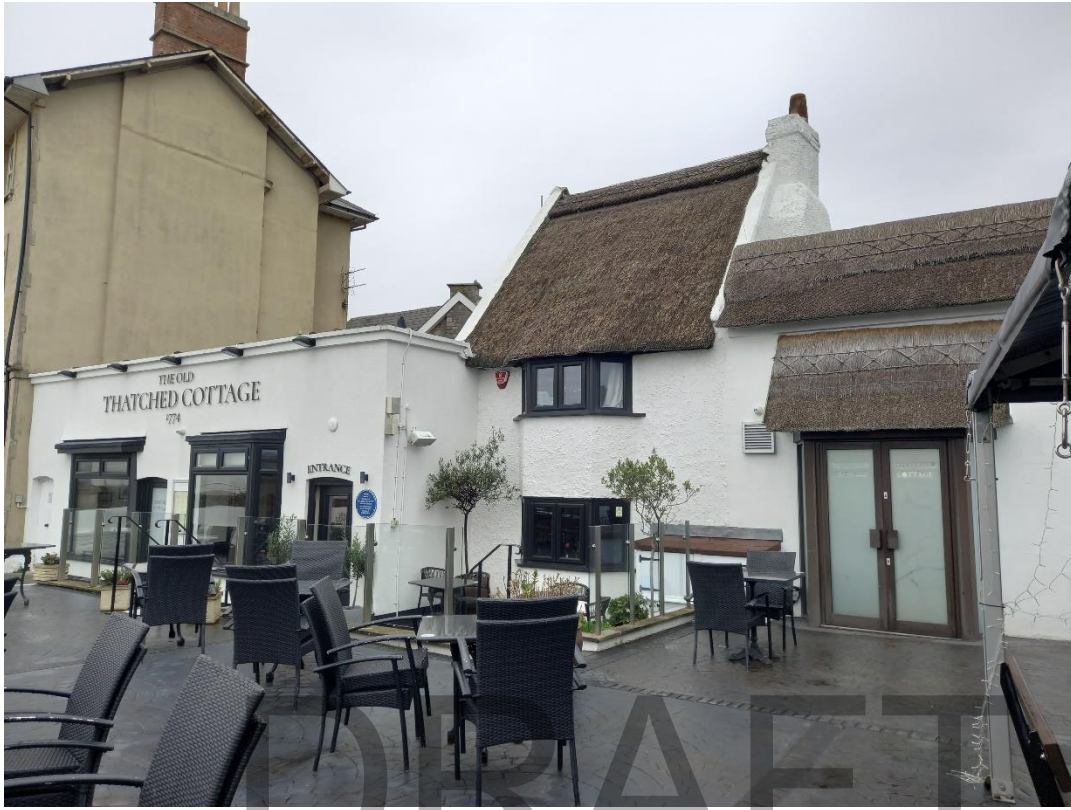
Plate 1 The Old Thatched Cottage Restaurant frontage (south elevation)
