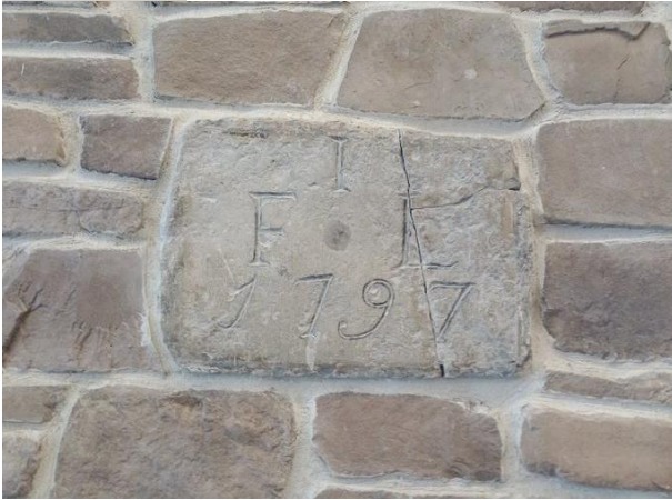
Plate 13. 1797 date stone in the wall of AB2
