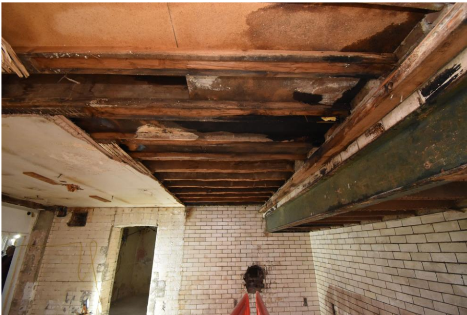
Photo 4.5: Ceiling in basement extension to 100 Church Road
