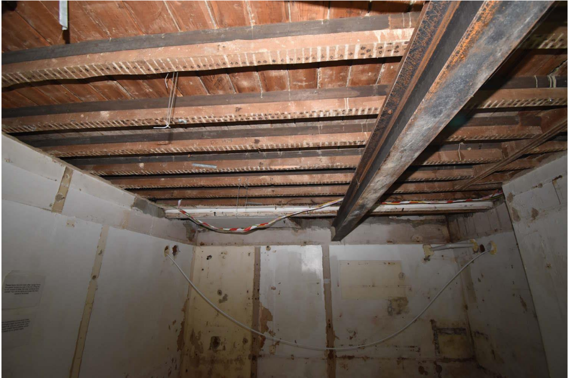
Photo 4.11: Underside of floor type B with additional steel support.
