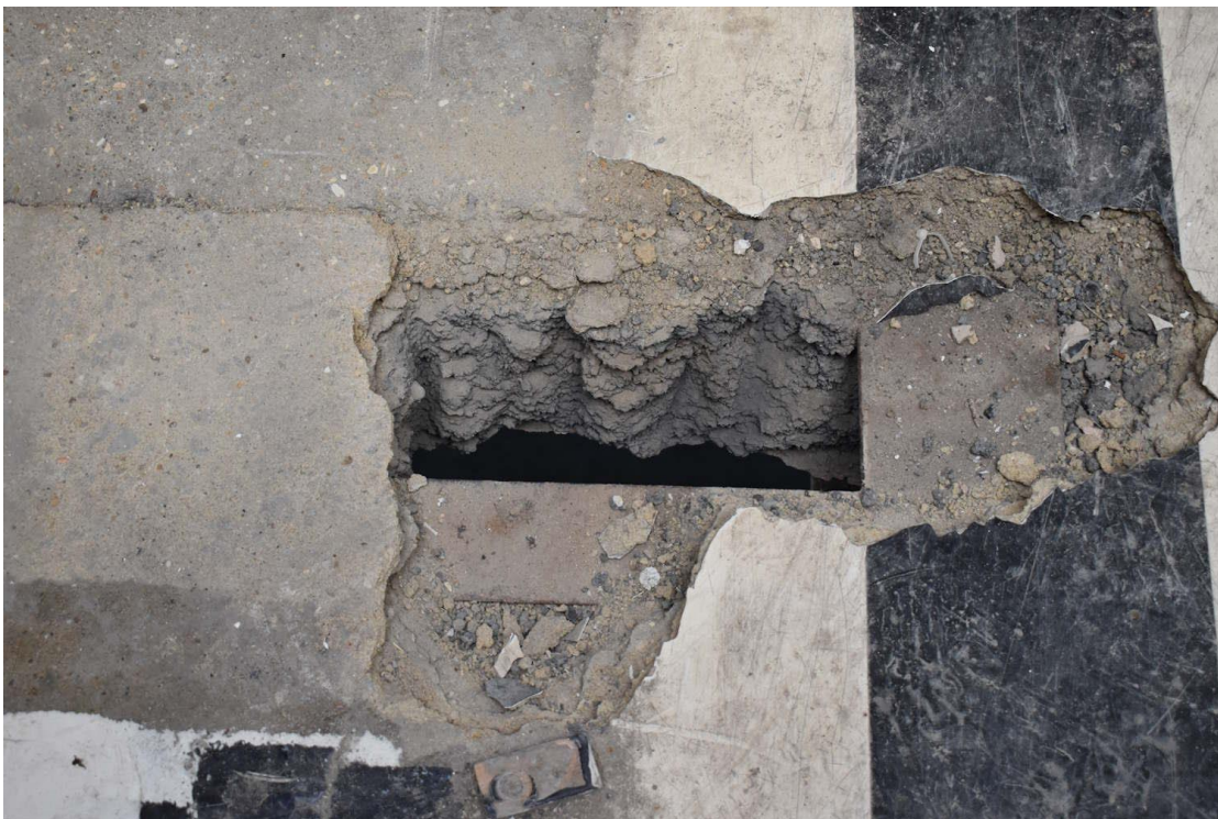
Photo 4.11: investigative hole into 'clinker' floor. Steel joists exposed. View from above.
