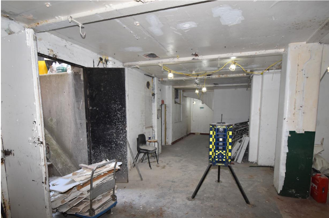
Photo 4.10: Basement extension of No.s 102 & 104. Ceiling of steel joists and cast 'Clinker'
