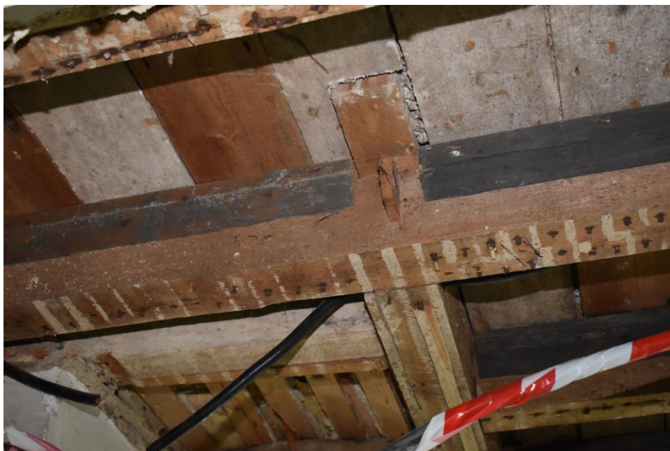
Photo 4.8: Adapted Floor Structure, viewed from below.
