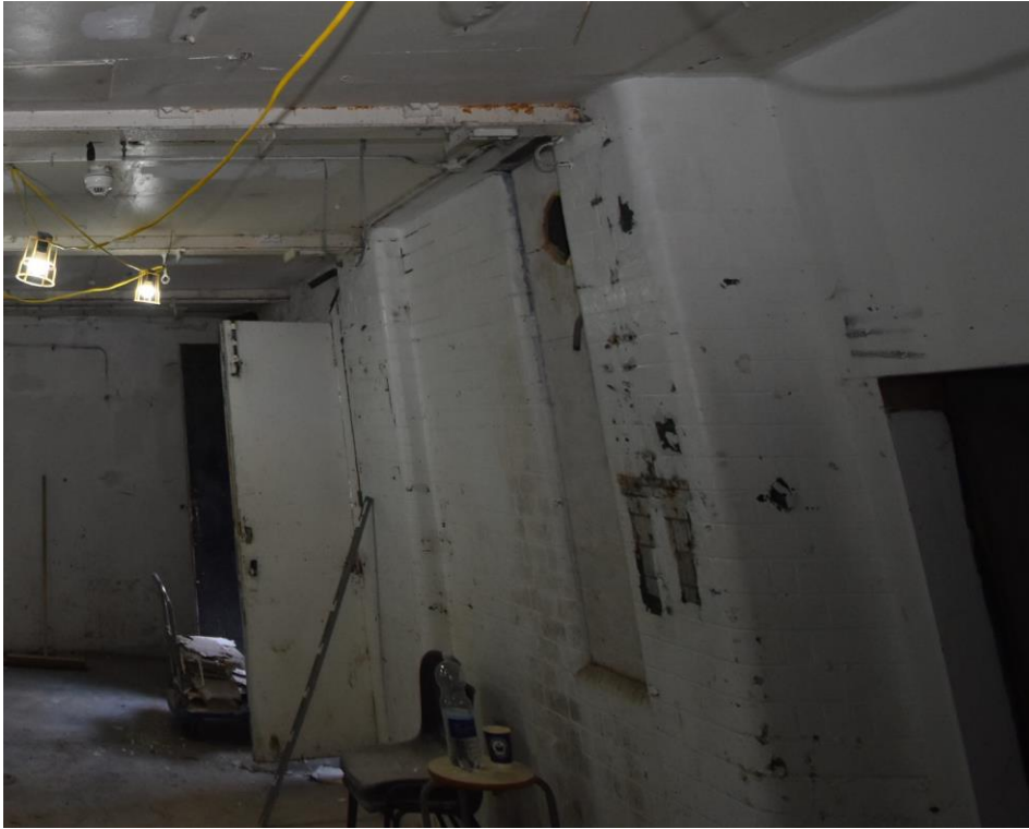
Photo 4.13: Narrow basement window, blocked internally
