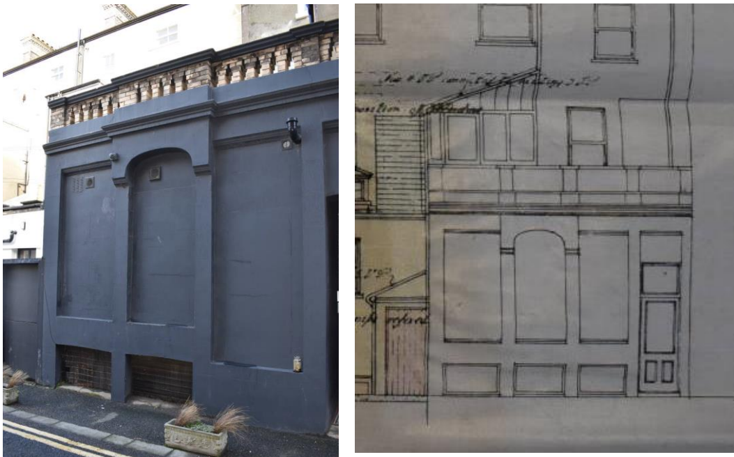
Figure 4.3: Rear of No. 100 Church Street, (right) elevation in c. 1911
