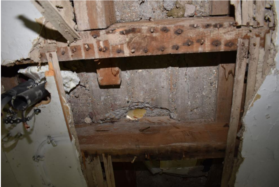
Photo 4.9: Underside of cast concrete floor – a section of floorboards removed.
