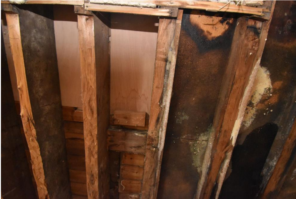
Photo 4.6: Detail of ceiling to basement extension in 100 Church Road
