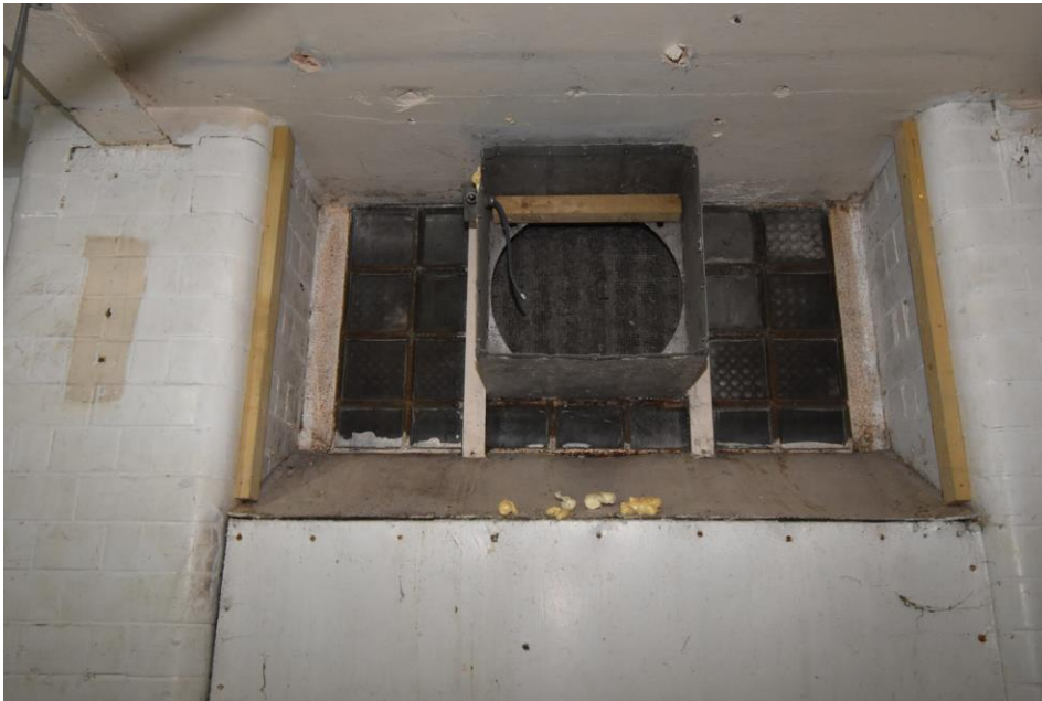
Photo 4.14: partially blocked wider basement window with existing vent
