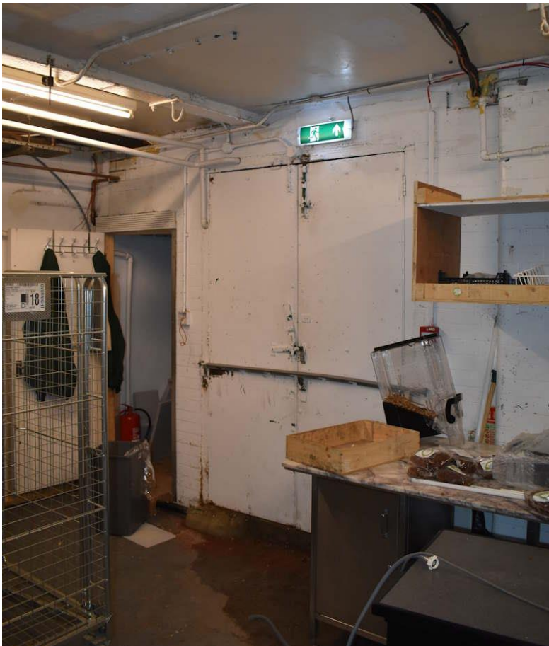
Photo 4.12: Modern rear basement double doors leading to rear yard
