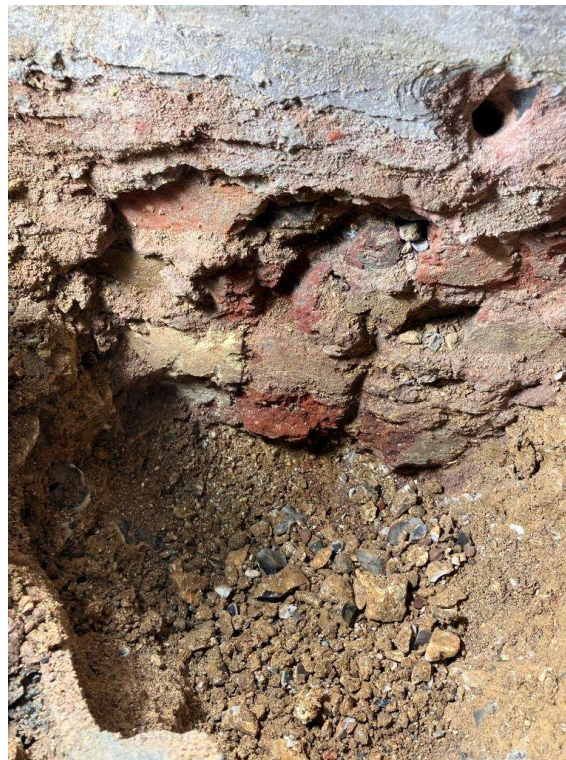
Figure 4 – Trial Pit Showing the Made-up Ground (Flint/Shingle)
