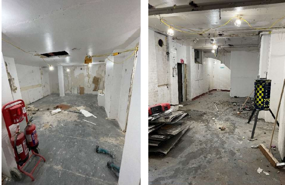
Figure 1 – Existing Basement Ground Slab
