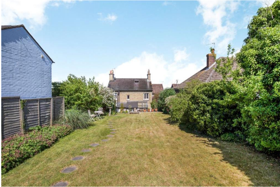
Rear Elevation viewed from the rear garden
