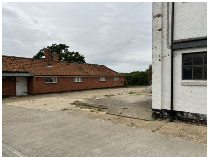
Image of the building to be renovated and extended, showing the ‘farmyard’ area
