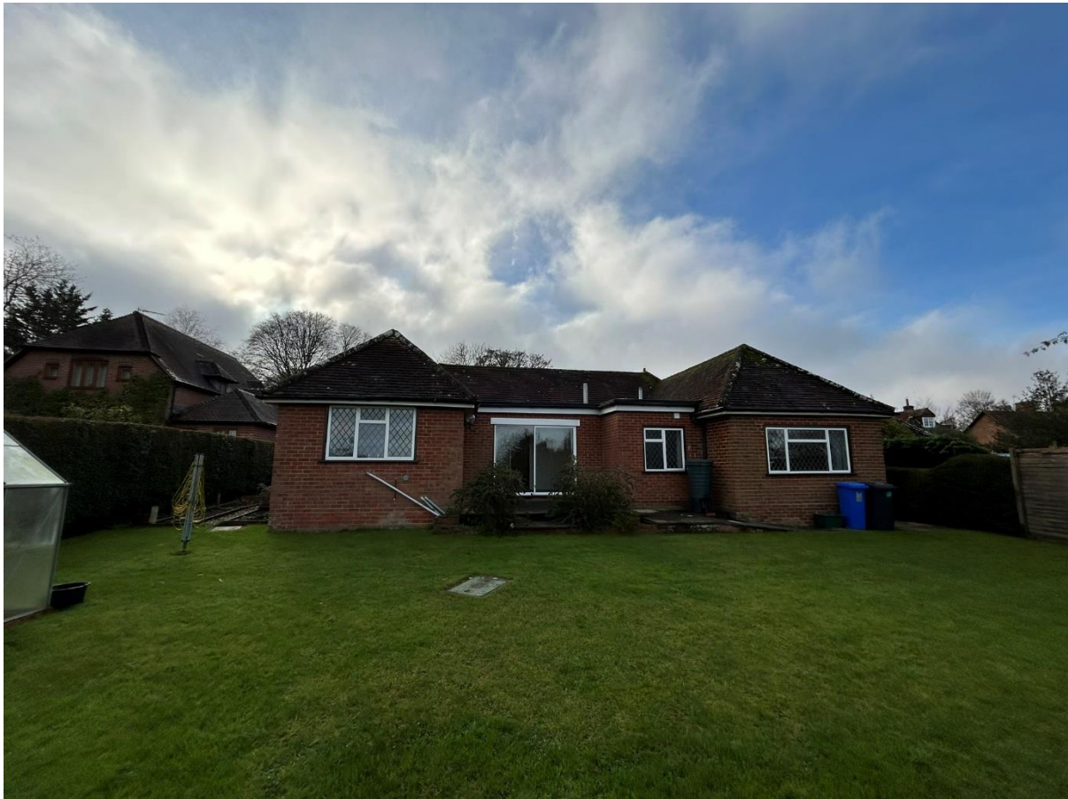
Fig. 1 – View of existing rear elevation
