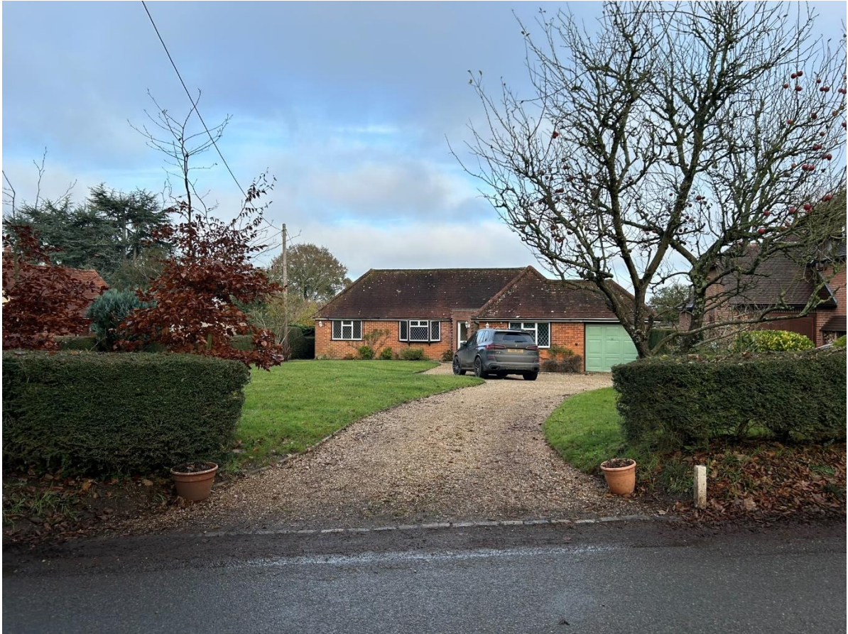
Fig. 2 – View of Little Copse from The Street
