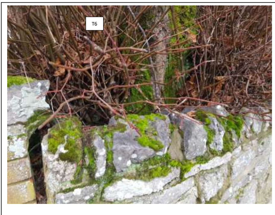
View of base of T6
