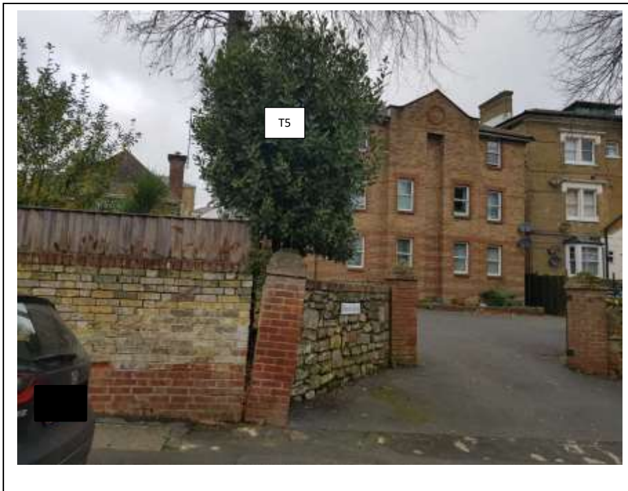
View of pier adjacent to T5
