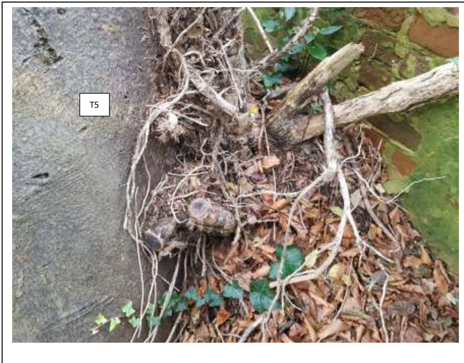
View of base of T5
