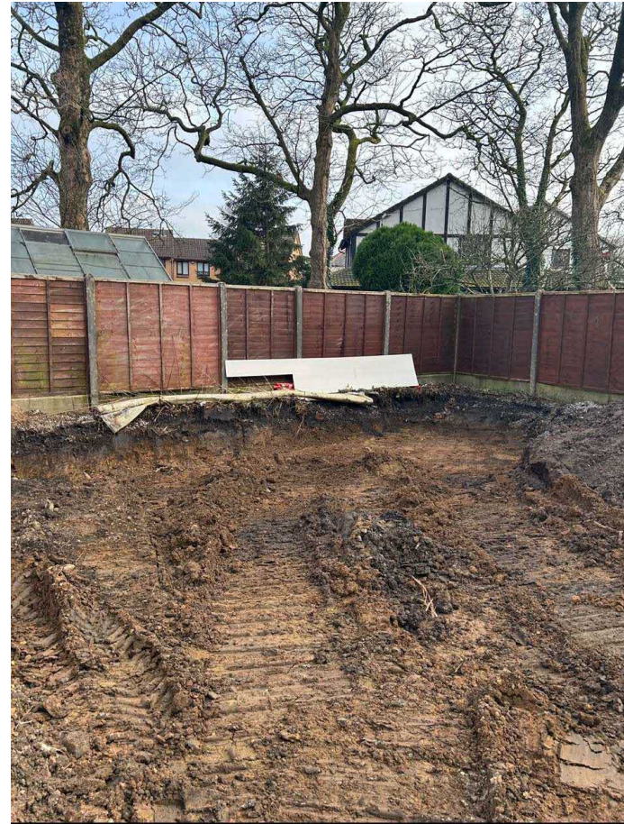
Stripped north eastern area.
