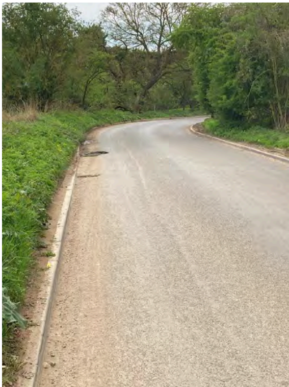
5.14 Past the first corner is a pothole on the southern side of the road which has developed, through the wearing course and sub-base.
