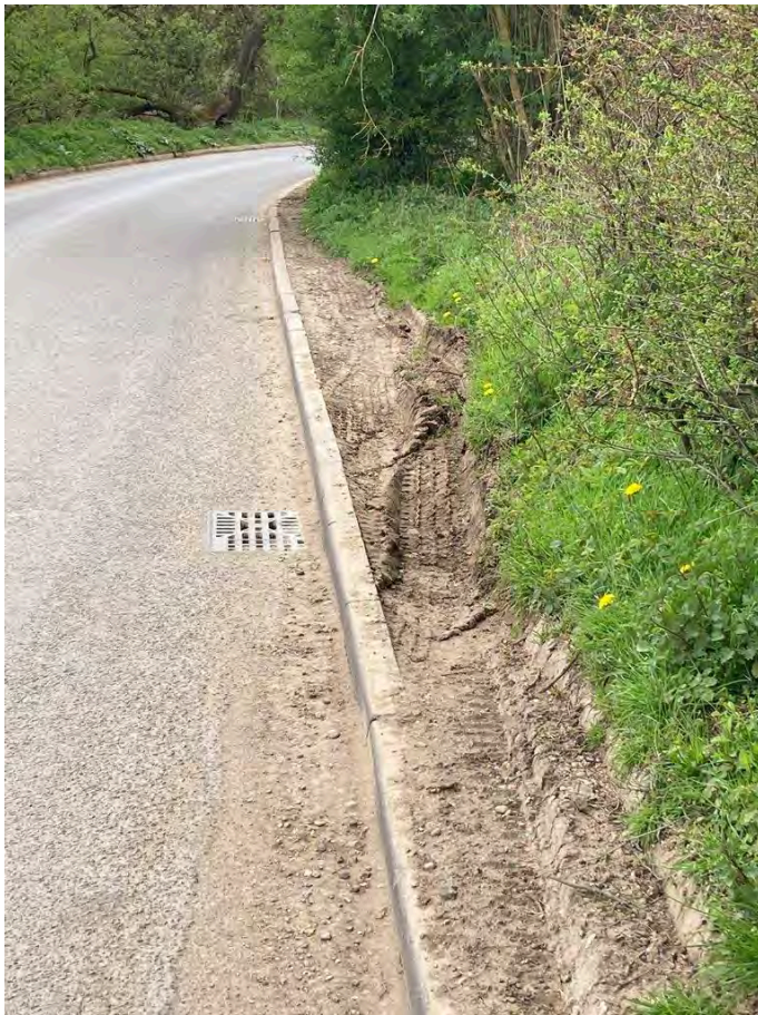
5.14 Past the first corner is a pothole on the southern side of the road which has developed, through the wearing course and sub-base.
