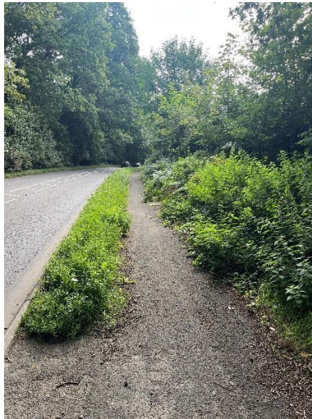
Photograph 6: Southern A36 Footway
