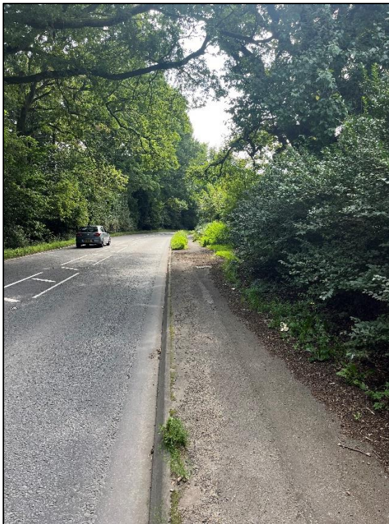
Photograph 21: Existing conditions on Salisbury Road (A36) after Hill Street Bus Stop
