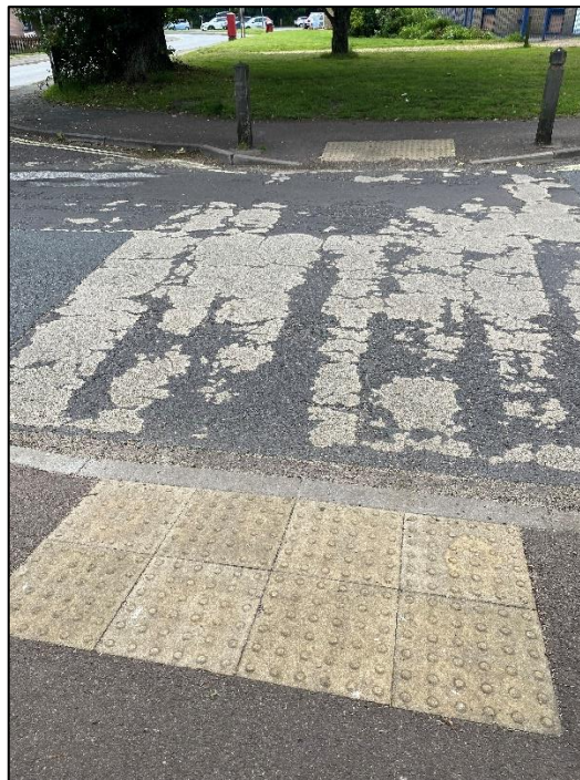
Photograph 15: Dropped kerb crossing with tactile paving across Calmore Drive
