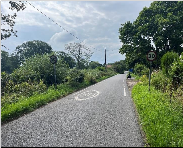
Photograph 3: Existing conditions along Pauletts Lane
