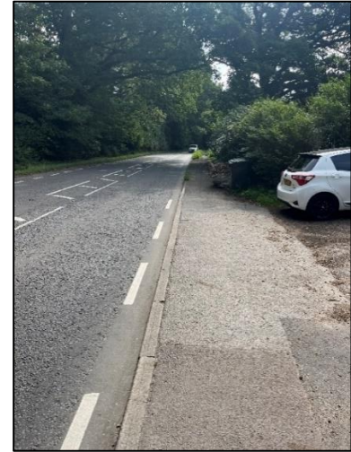
Photograph 20: Existing conditions on Salisbury Road (A36) after Hill Street Bus Stop
