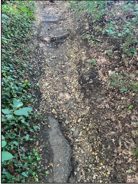
Photograph 16: Footway from Pauletts Lane to Hill Street Bus Stop
