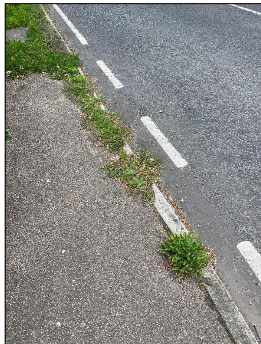
Photograph 9: Dropped kerb crossing at Calmore Road
