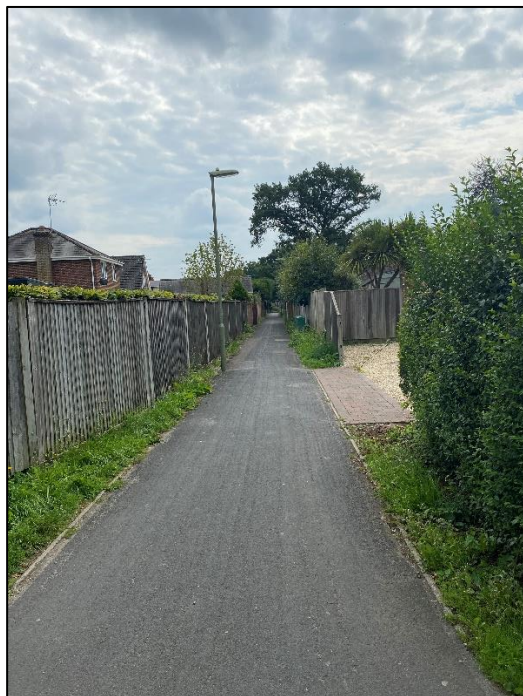
Photograph 12: Conditions on footpath from Calmore Road to Calmore Drive
