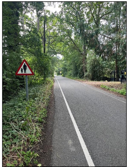
Photograph 6: Existing conditions along Pauletts Lane
