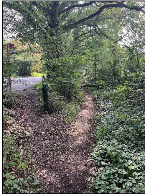
Photograph 18: Footway from Pauletts Lane to Hill Street Bus Stop
