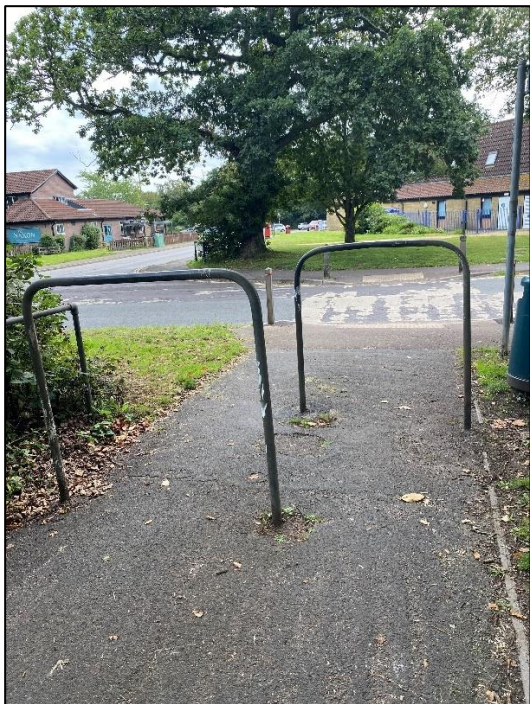
Photograph 14: Conditions on footpath from Calmore Road to Calmore Drive
