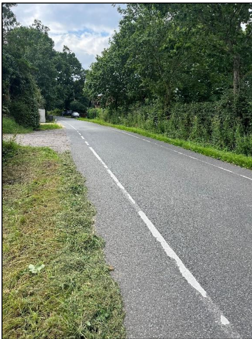
Photograph 5: Existing conditions along Pauletts Lane
