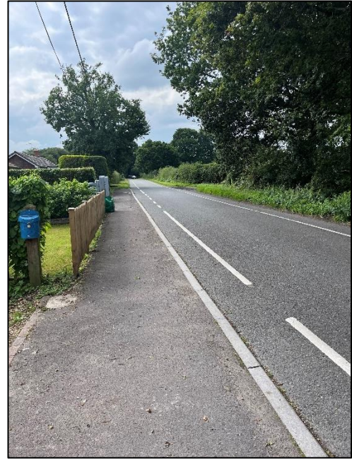
Photograph 4: Existing conditions along Pauletts Lane
