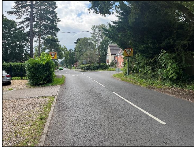
Photograph 7: Existing conditions along Pauletts Lane
