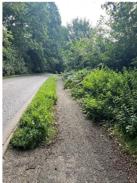
Photograph 6: Southern A36 Footway
