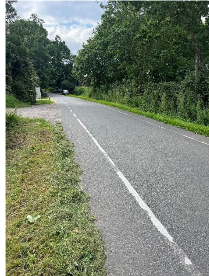
Photographs 4 and 5: Pauletts Lane Conditions
