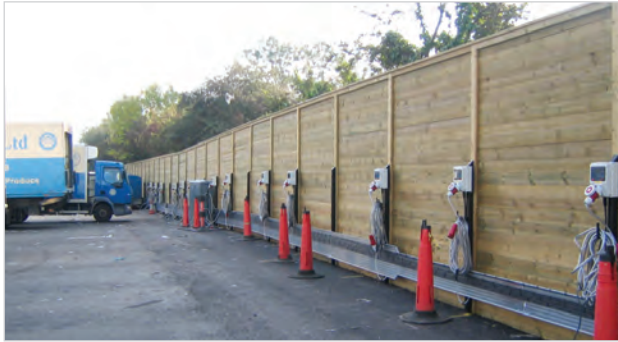
Grimshaw Kinnear - 100m of 3m high Jakoustic fencing
