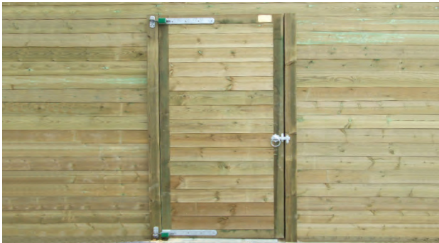
2m high x 1m wide gate within 3m high Jakoustic fencing
