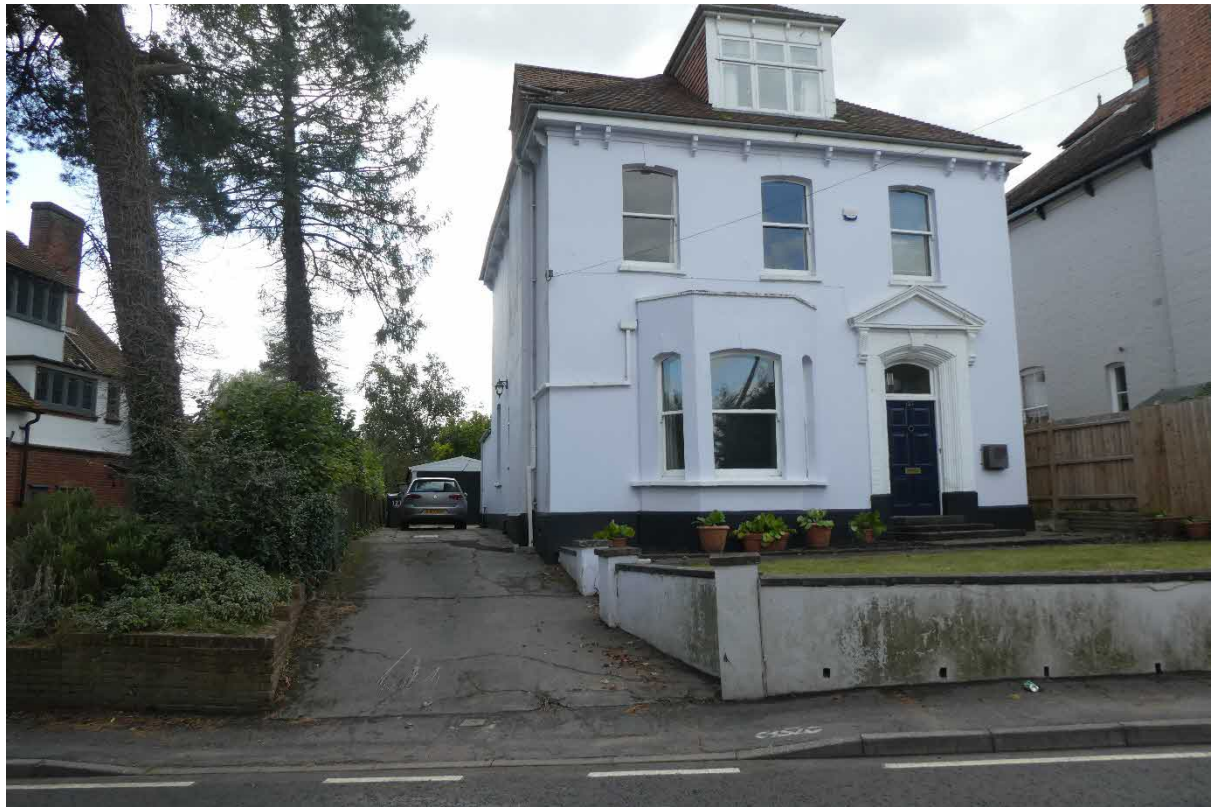
127 Hadham Road, CM23 2QD: photographs taken after work on garage roof completed
