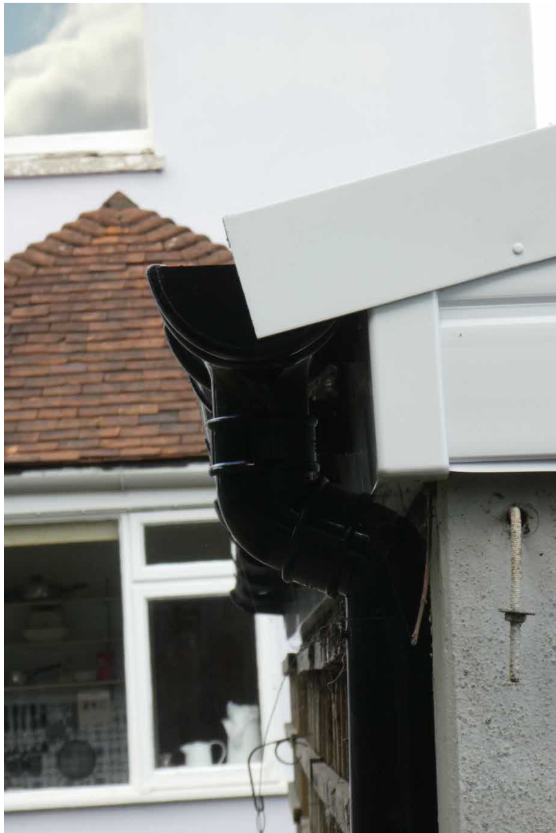
127 Hadham Road, CM23 2QD: photographs taken after work on garage roof completed
