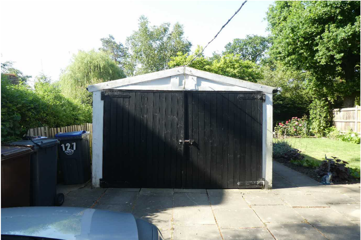
Front of Garage showing detail of leading edge of roof.
