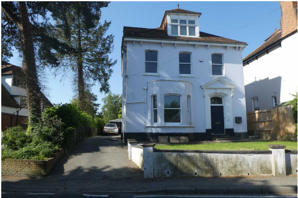
Garage as seen from public highway (far side of road)
