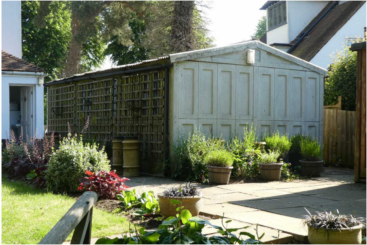
Garage from back garden – close up showing details of construction
