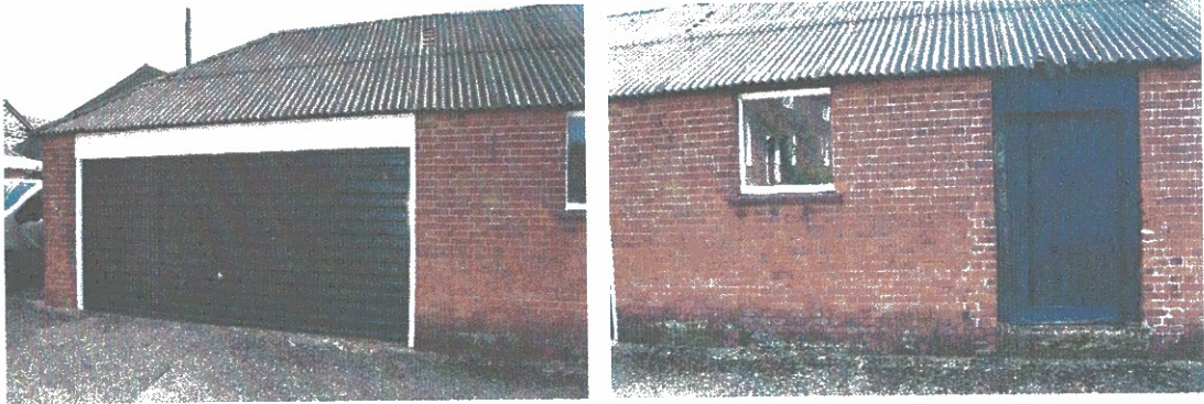
Plates 10 and 11: South outbuilding, west elevation
