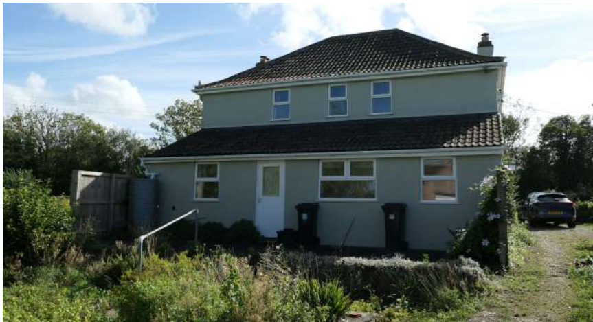
Rear north facing elevation.
