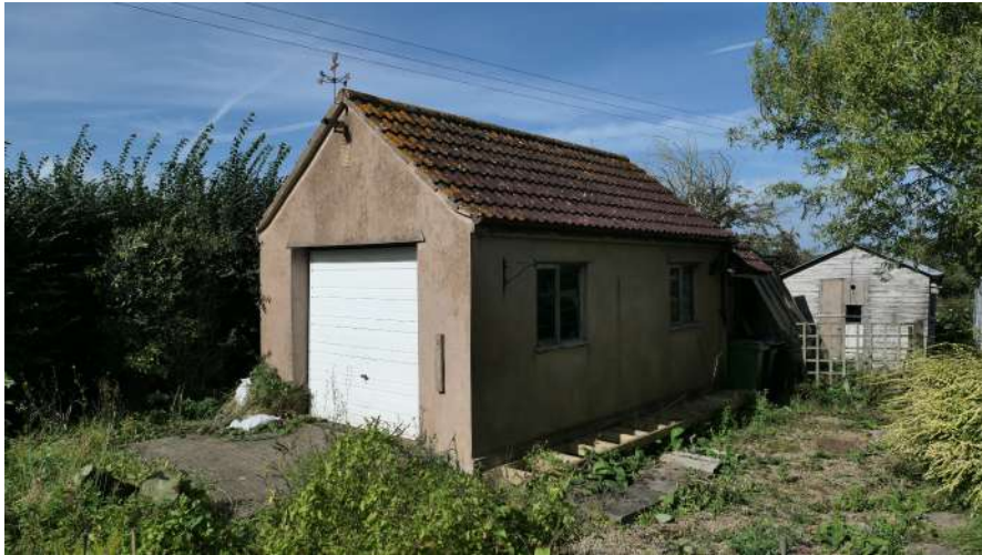
View 2 - Garage and shed outbuildings along west boundary to north end.
