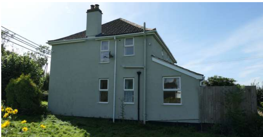
South west elevation facing towards paddock site.
