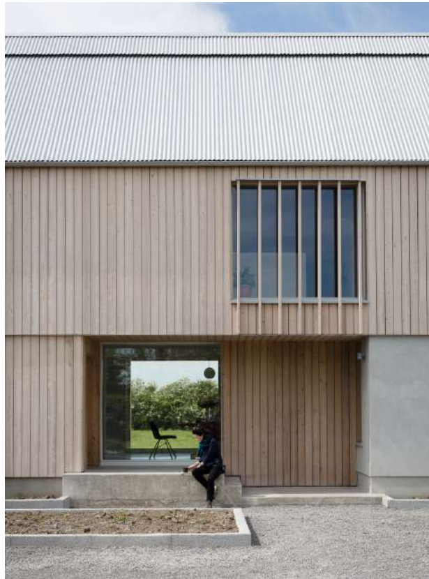
Example of pale natural timber cladding with light grey corrugated metal roofing.
