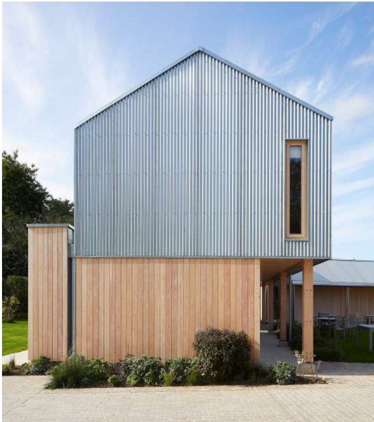
Example of silvery corrugated metal cladding to upper storey over timber clad ground floor.
