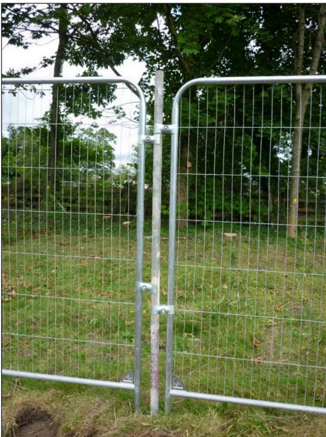
Tree Protective Fencing Specification
